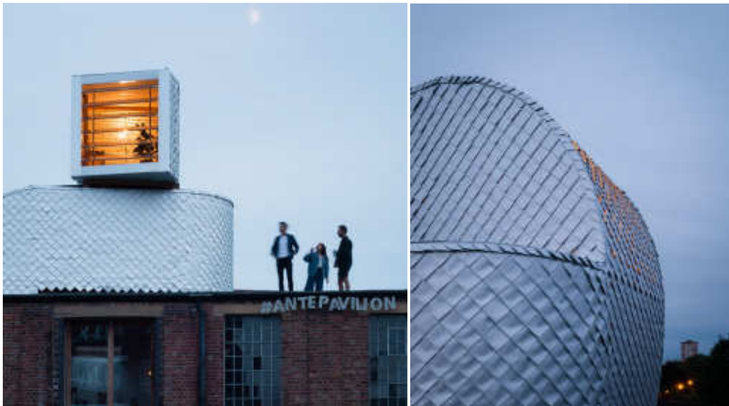
Figura 33: Intervenção parasita Antepavilion - warehouse air duct (Fonte: https://www.dezeen.com/2017/08/04/pup-architects-roof-pavilion-antepavilion-air-duct-architecture-foundation-shiva-london-hackney/ , consultado em: out/2018).
