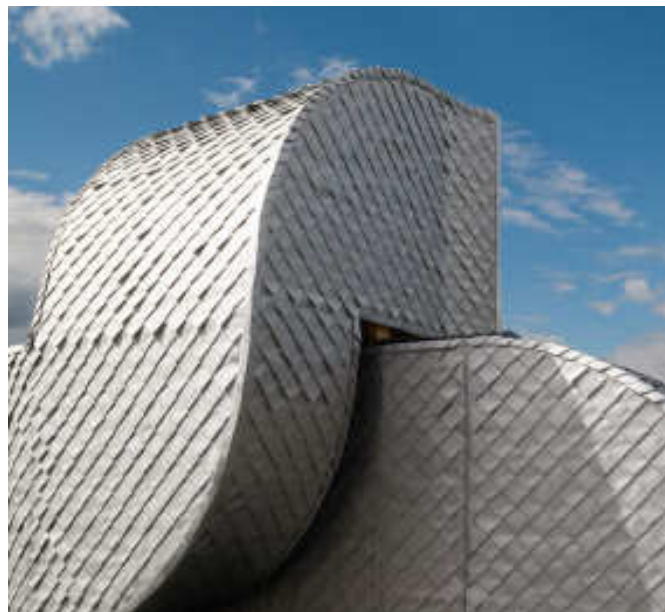
Figura 34: Intervenção parasita Antepavilion - warehouse air duct (Fonte: https://www.dezeen.com/2017/08/04/pup-architects-roof-pavilion-antepavilion-air-duct-architecture-foundation-shiva-london-hackney/ , consultado em: out/2018).
