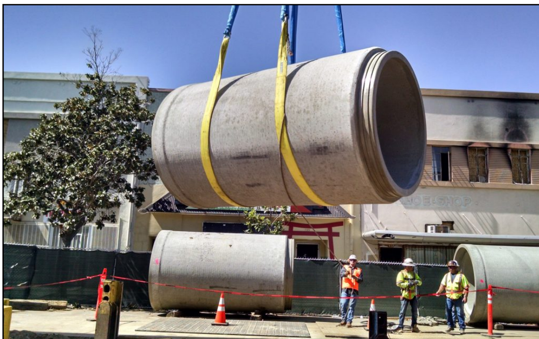
Figure 19. Utility Relocation for the HSR Project
