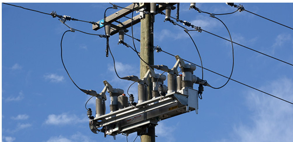
Figure 1 S&C IntelliRupter ® PulseCloser ® Fault Interrupter [1]
