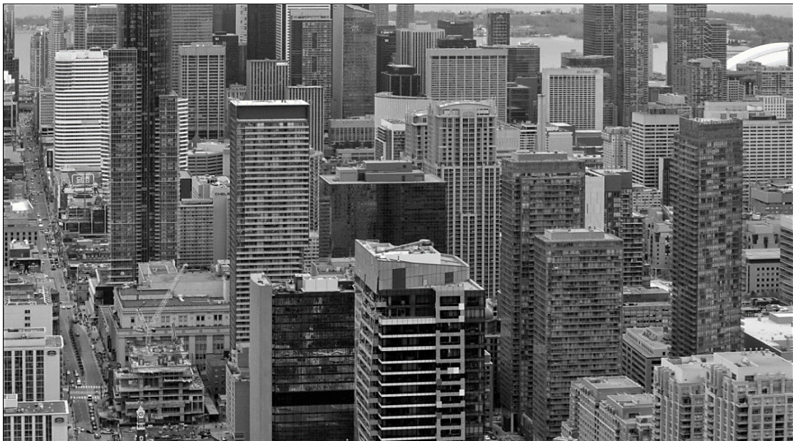
Figure 3-1: High-rise buildings with interacted façade system, Toronto
