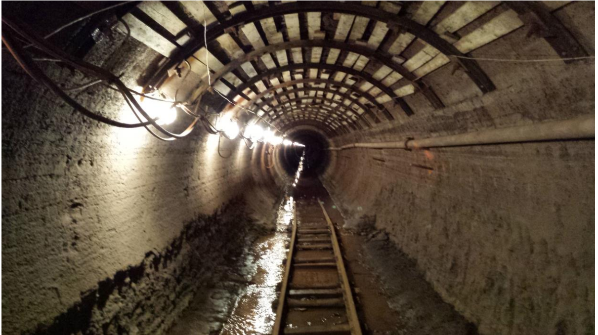
Figure 5.2. Excavated tunnel showing the McNally support system.
