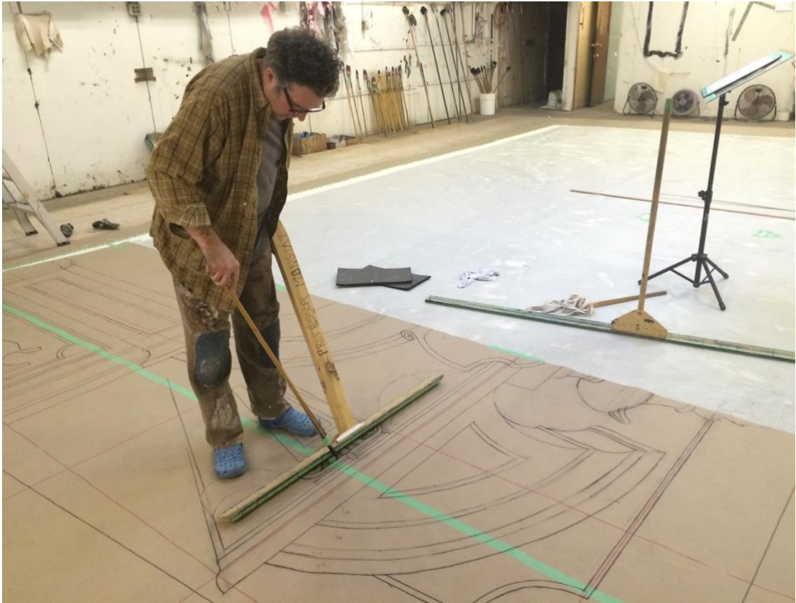
Figure 4.6: Lucio Silla. Designer Gerard Gauci and scenic artist Richard Mongiat. Here Richard is scaling up a drawing using a grid.
