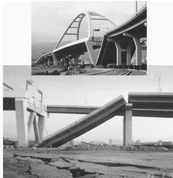
Figure 1.1: Nishinomiya-ko Bridge collapse in the 1995 Kobe earthquake in Japan (Moehle and Eberhard 2000)
