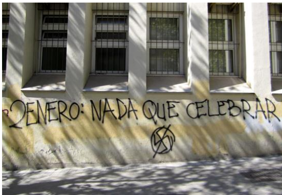
Figure 4.14: Graffiti written on the back of a public building echoes slogans of critics of the Día de la Toma , declaring “2 nd of January: Nothing to celebrate” (24 September, 2011; photo by author)
