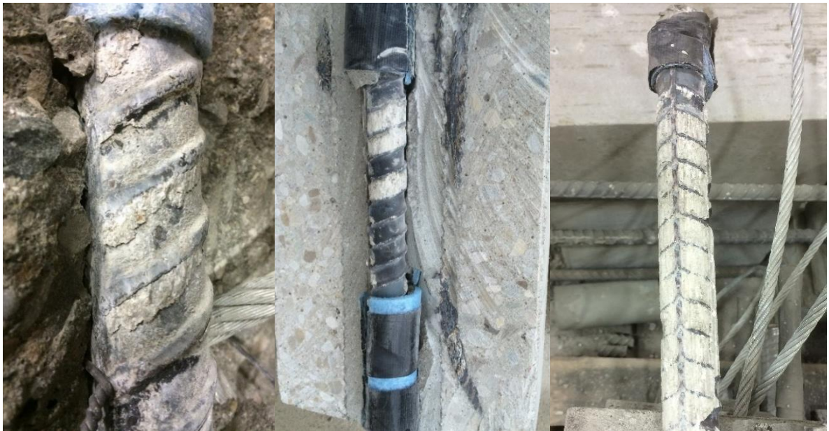
Figure 4.7: (left to right) Wedging of grout keys between ribs in a (C-6-D2); and Crushing of grout keys between ribs at 6 and 10 db embedment (NS-6-D1 and NS-10-D2, respectively).
