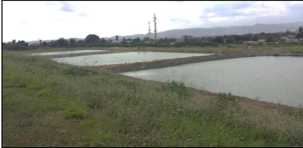
Figure 3.4 Side of the Legon Waste Stabilization Ponds in Accra (showing maturation ponds).
