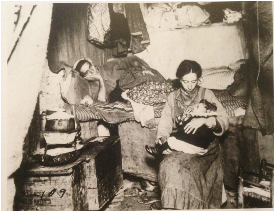
Figure 22: “Corner in basement of ruined building where nine persons (2 families) live in one corner. Saloniki, Greece” (GCAH-79372)
