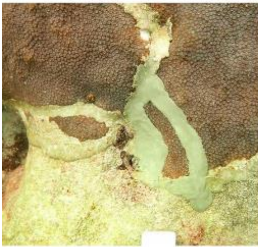
June 1, 2018- Addition of FB and more epoxy on margin
