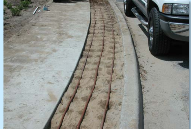
Installing micro-irrigation to avoid waste
