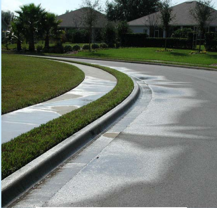
Too much water wasted
