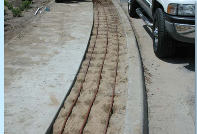
Installing micro-irrigation to avoid waste
