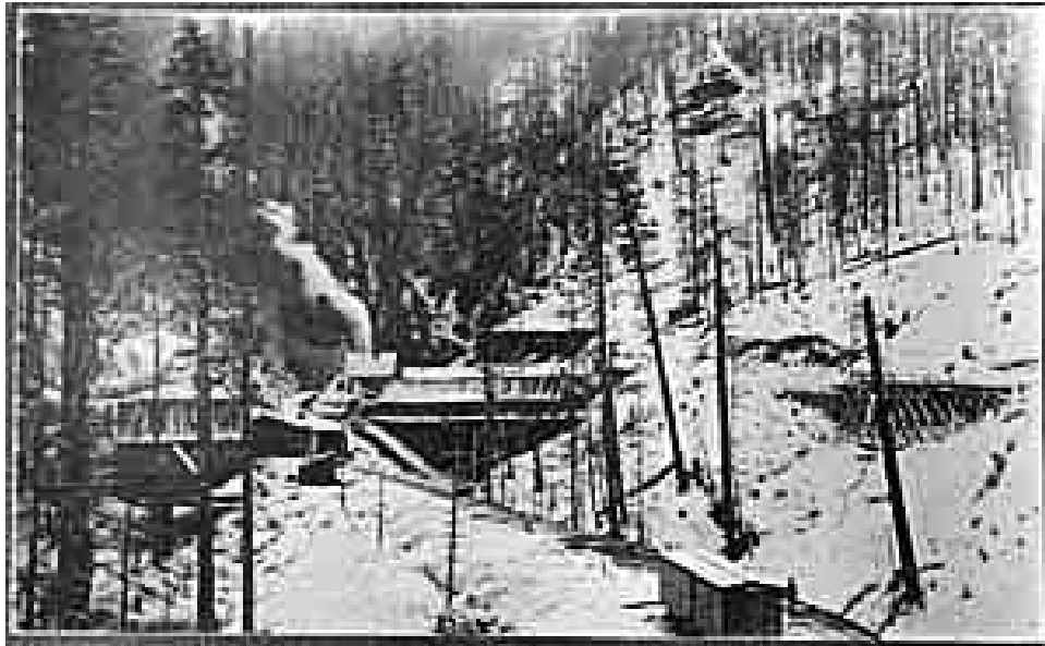
East Portal of Northern Pacific's Stampede Pass Tunnel known as Martin.
