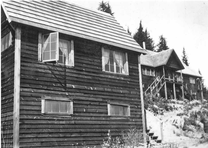
Martin, caretaker's cabin in foreground and ski hut in background. Courtesy of Northern Pacific Railway Historical Association, Jim Fredrickson collection.
