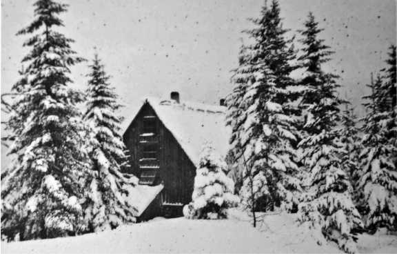
Meany Ski lodge, 1929, courtesy of The Mountaineers.
