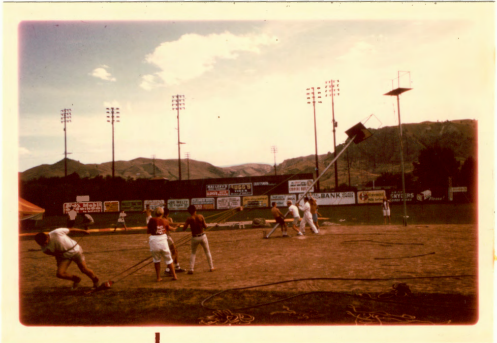
Figure 14. Hoisting high wire pedestal into air.
