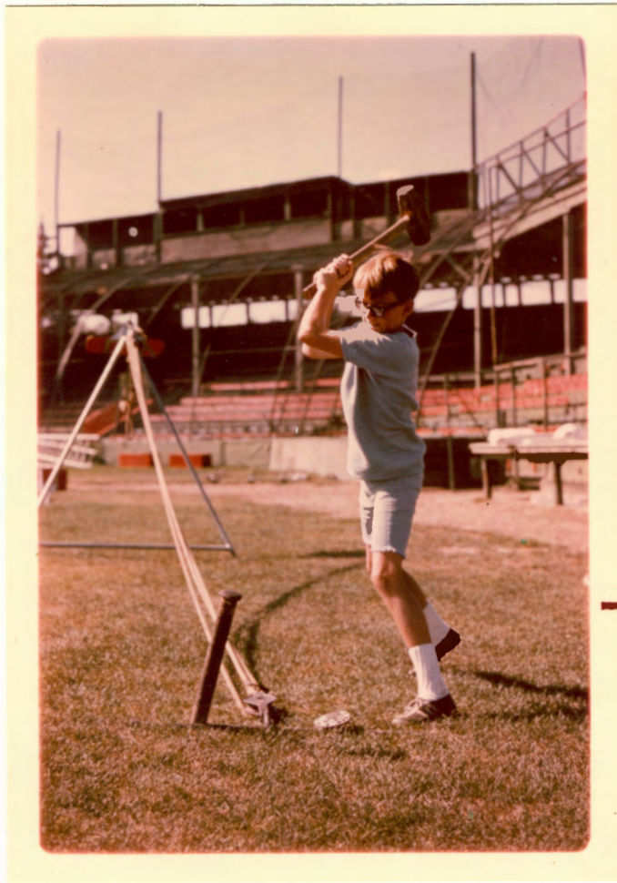
Figure 9. Guying tight wire.
