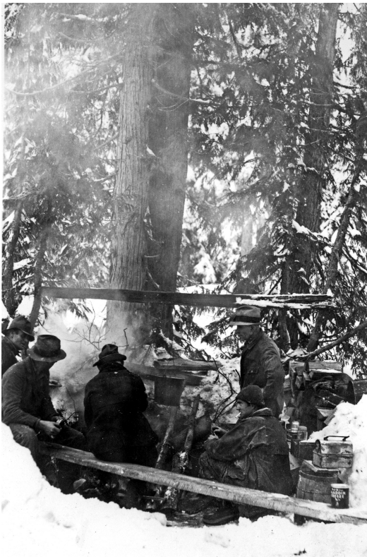
Work on Seattle Ski Park, December 1933, Seattle Photo archives, # 31172.
