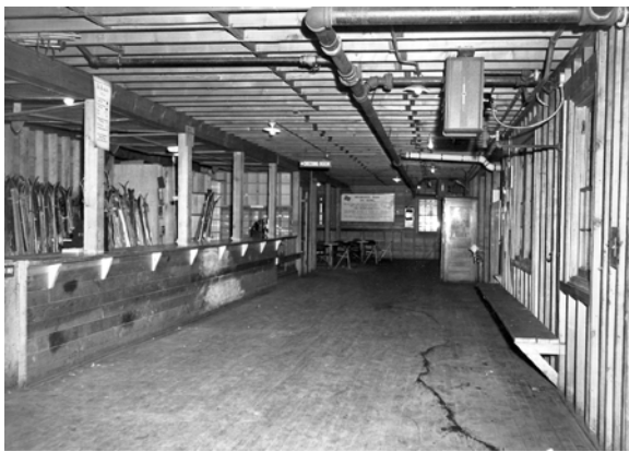
Ski room on first floor. Courtesy of Walter Page.
