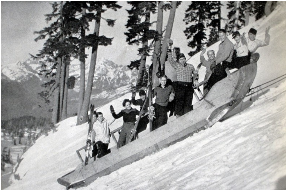
Mount Baker ski escalator, January 1936. Picture courtesy of Kirby Gilbert.
