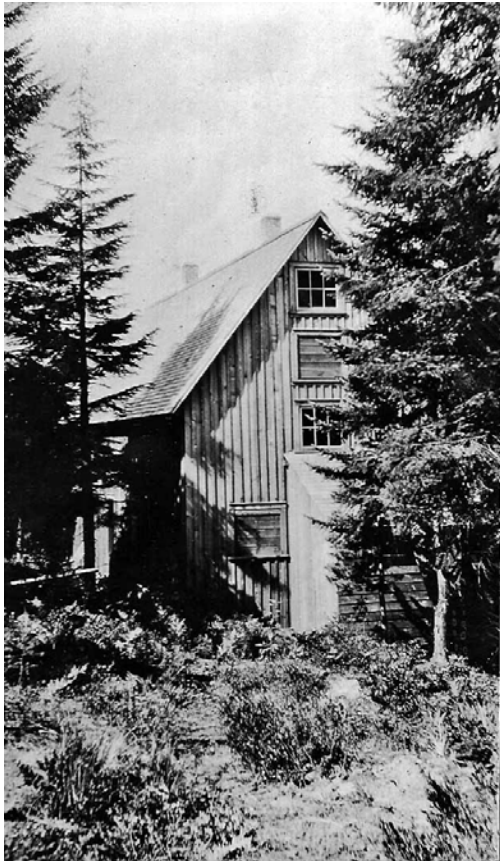
Meany Lodge, 1930s, Mountaineers' photo by Bob Sterling
