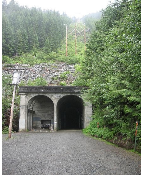
West Portal of Milwaukee RR tunnel, the old Rockdale stop.
