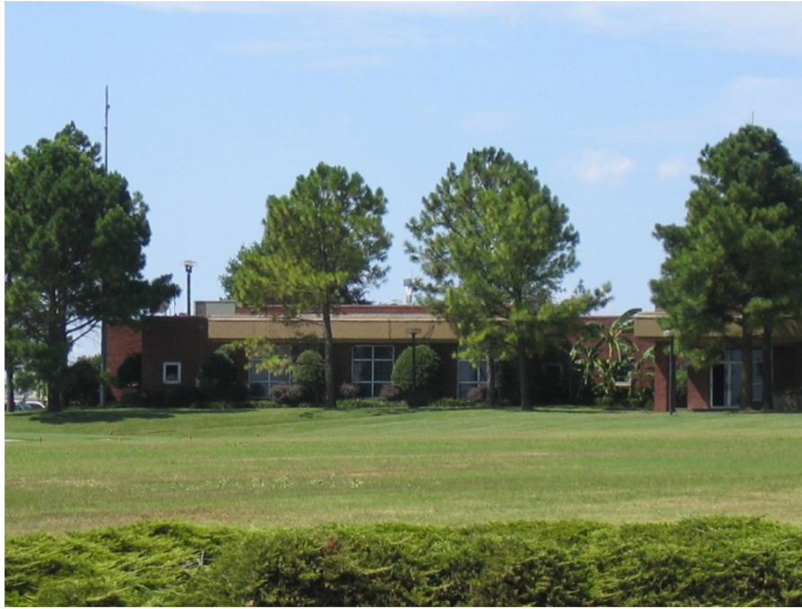
Figure 9-5. The Port Headquarters building with network node on the roof.
