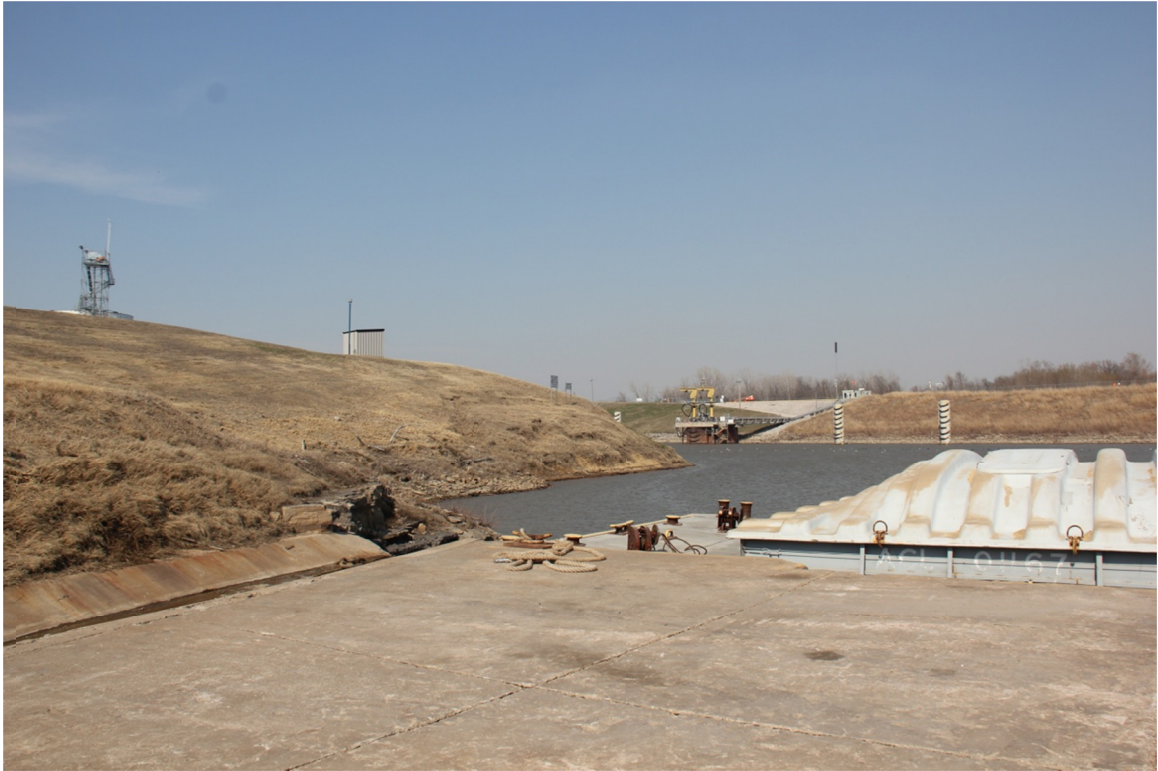
Figure 9-7. Location of the PTZ camera installation at the entrance to the port.
