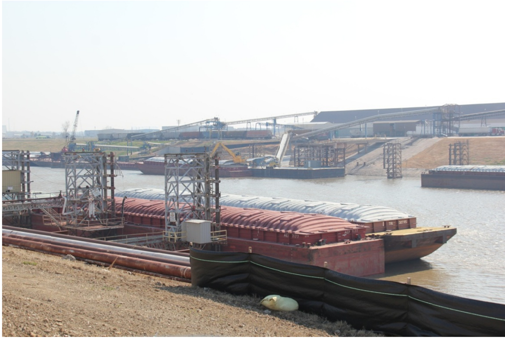
Figure 3-18. East Dry Bulk Terminal at the Port of Catoosa.
