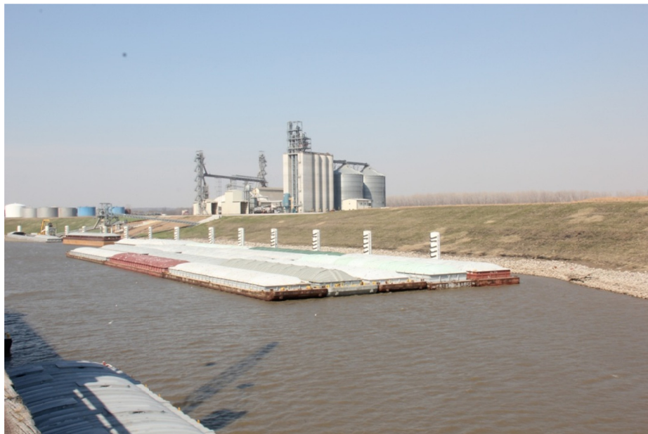
Figure 3-17. Grain Elevators at the Port of Catoosa.
