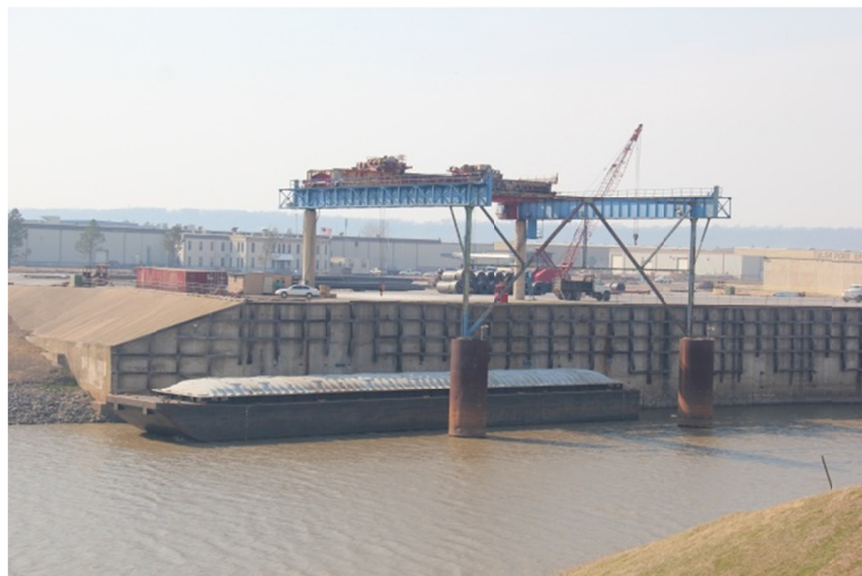
Figure 3-13. Overhead Travelling Bridge Crane.
