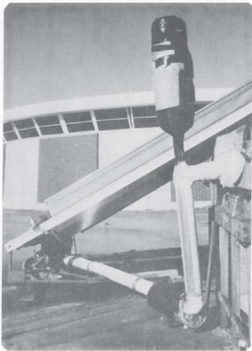
Fig. 4.6. Left side : Insulated pipe from heat exchanger to the pump.
