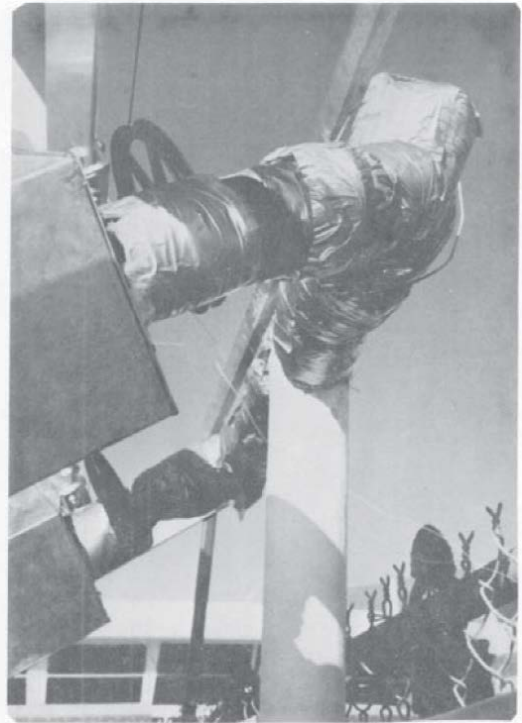
Fig. 4.10. Left side : Outlet end of heat exchanger, where the top surface and the edges were covered with fiberglass board insulation. The expansion tank as shown was also well insulated with fiberglass sheet.
