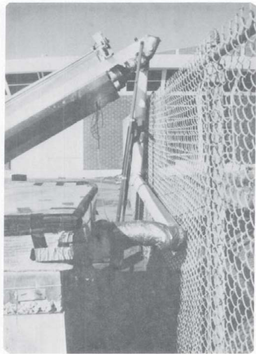
Fig. 4.6. Left side : Insulated pipe from heat exchanger to the pump.
