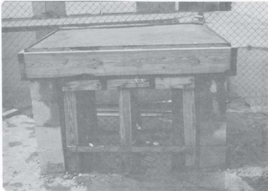
Fig. 4.4. After concrete was poured on forms and surface being levelled.
