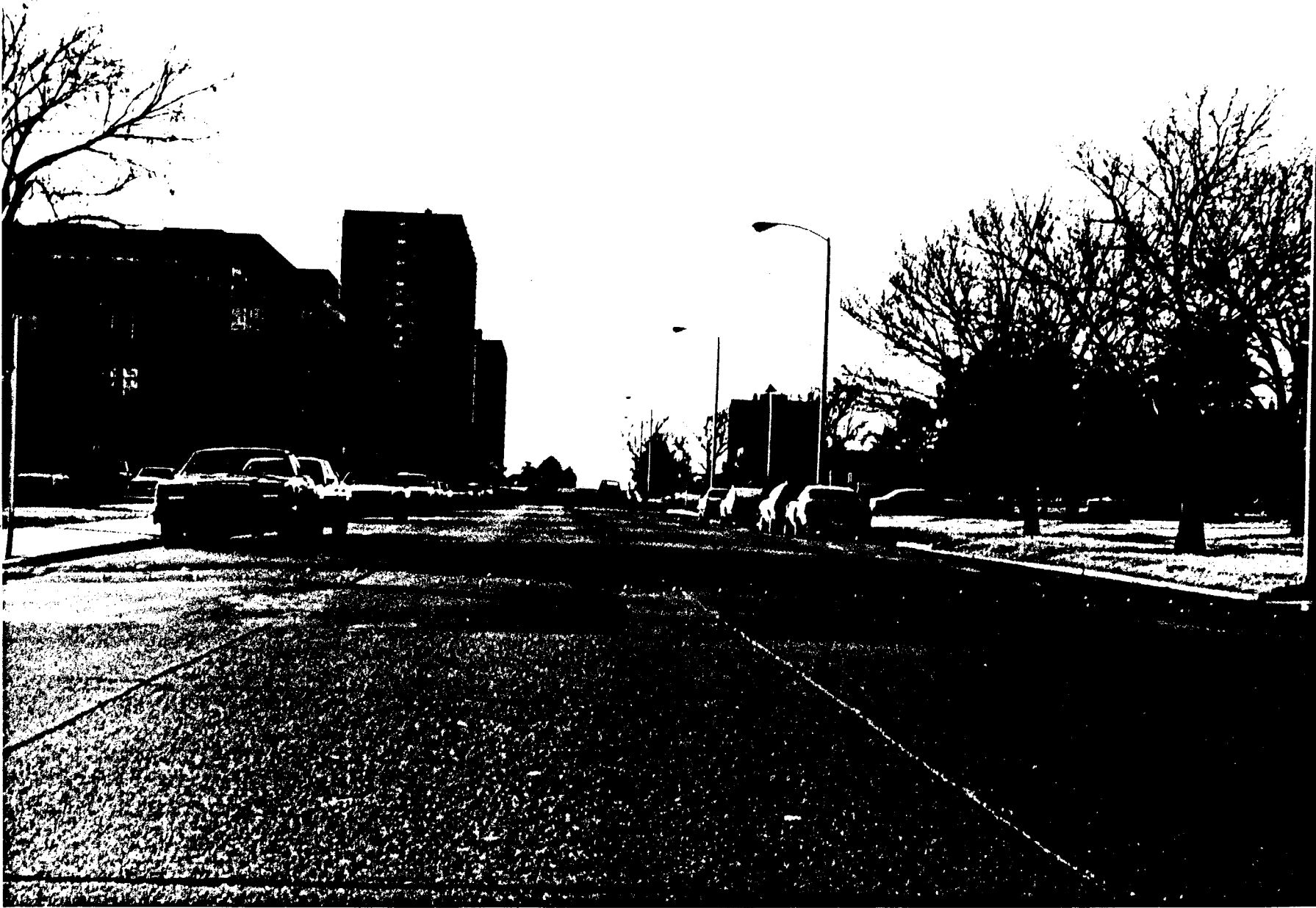
8) View looking west down Farm Road
