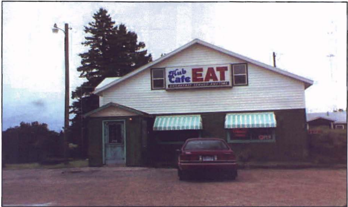
Figure 13. The Hub Cafe is a green metal building with white vinyl siding covering the upstairs living quarters. This restaurant is on US 41.
