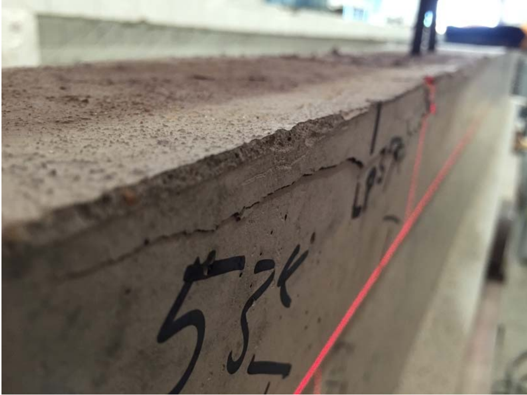
Figure 63. Concrete failure at top of top flange, C3NC
