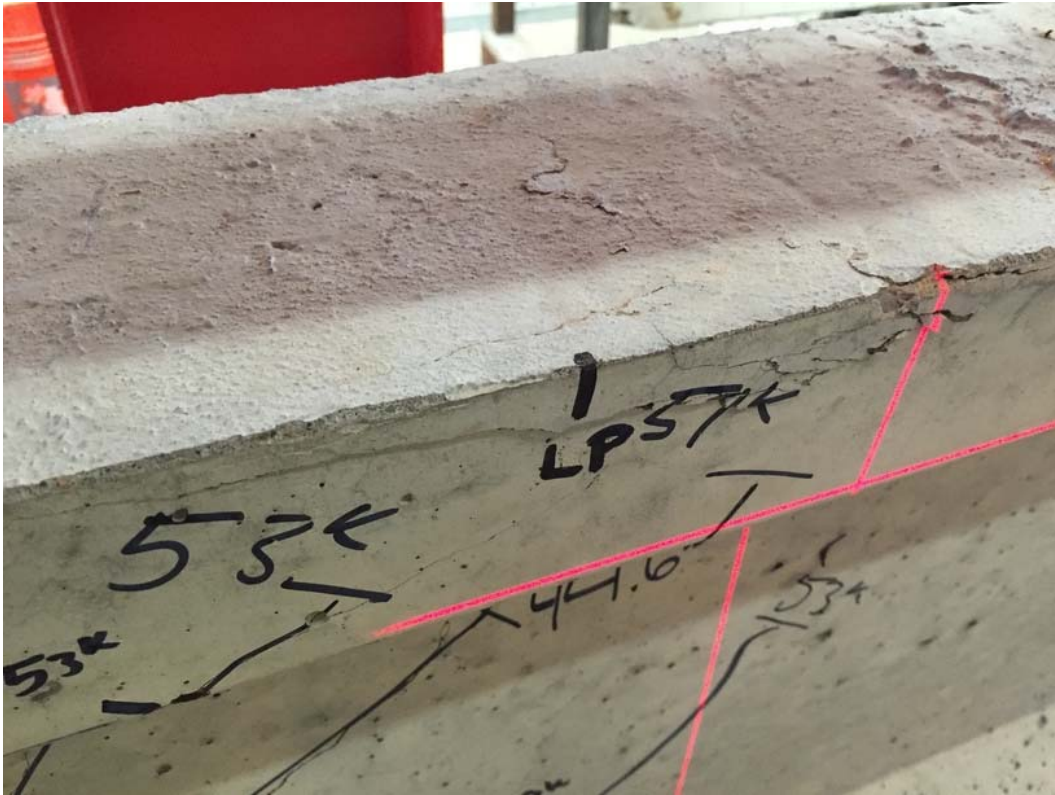
Figure 62. Concrete failure at top of top flange, C3NC
