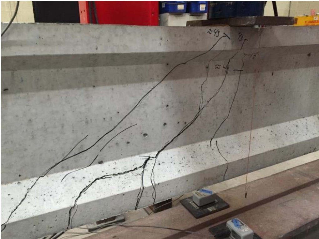
Figure 27. Visual Map of Cracking for Shear Test on A4N
