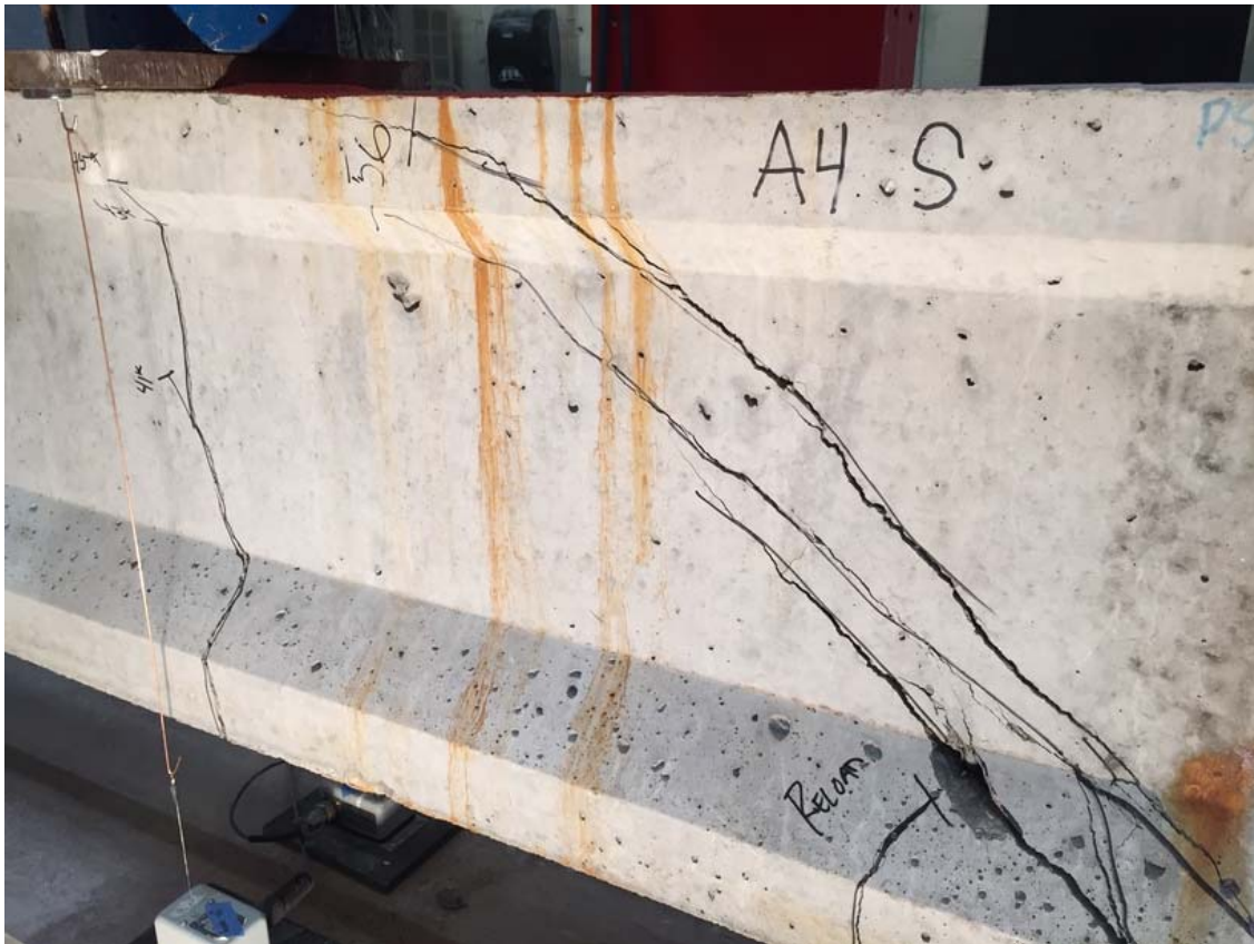
Figure 23. Visual Map of Cracking for Shear Test on A4SC
