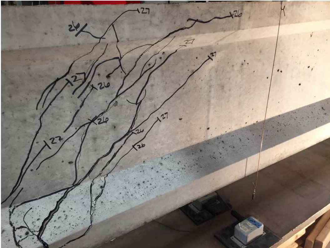
Figure 66. Visual map of cracking of C3S
