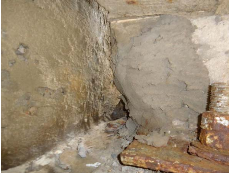
Figure 117. Repair to spalled back corner (6N-W)
