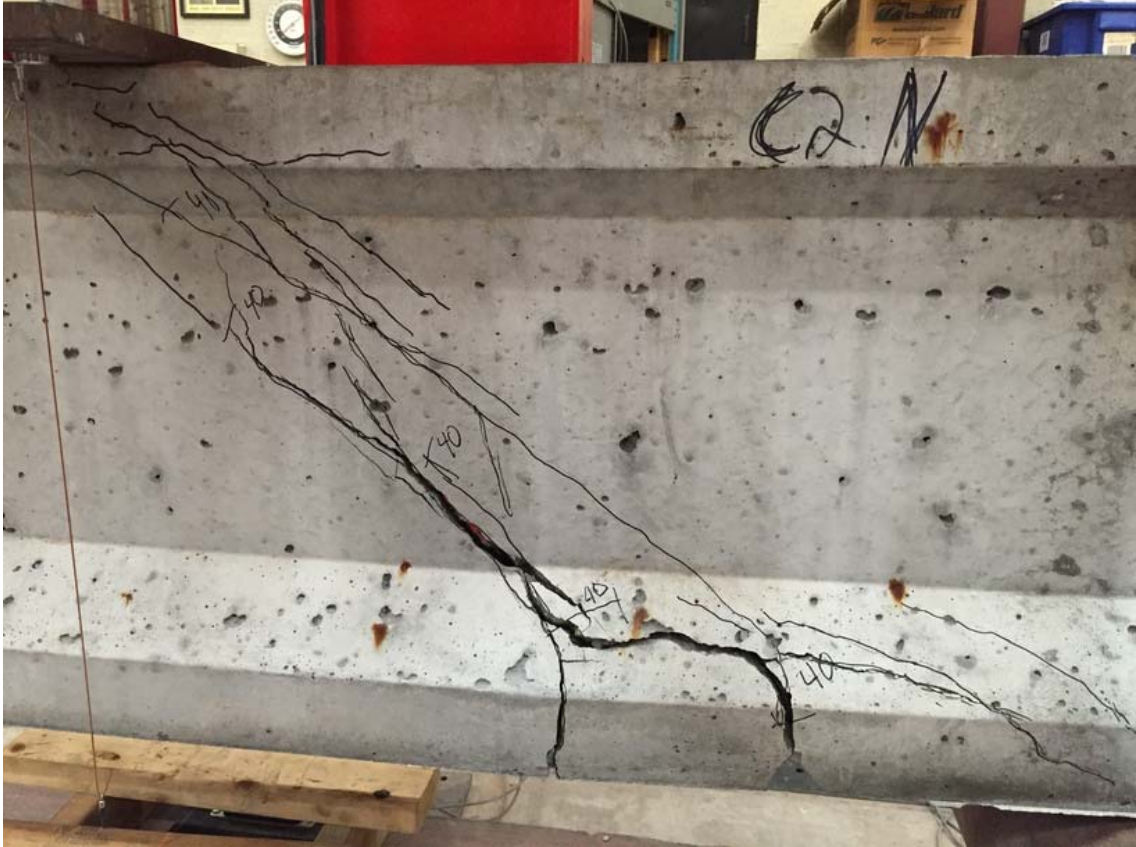
Figure 52. Visual Map of cracking of C2NC
