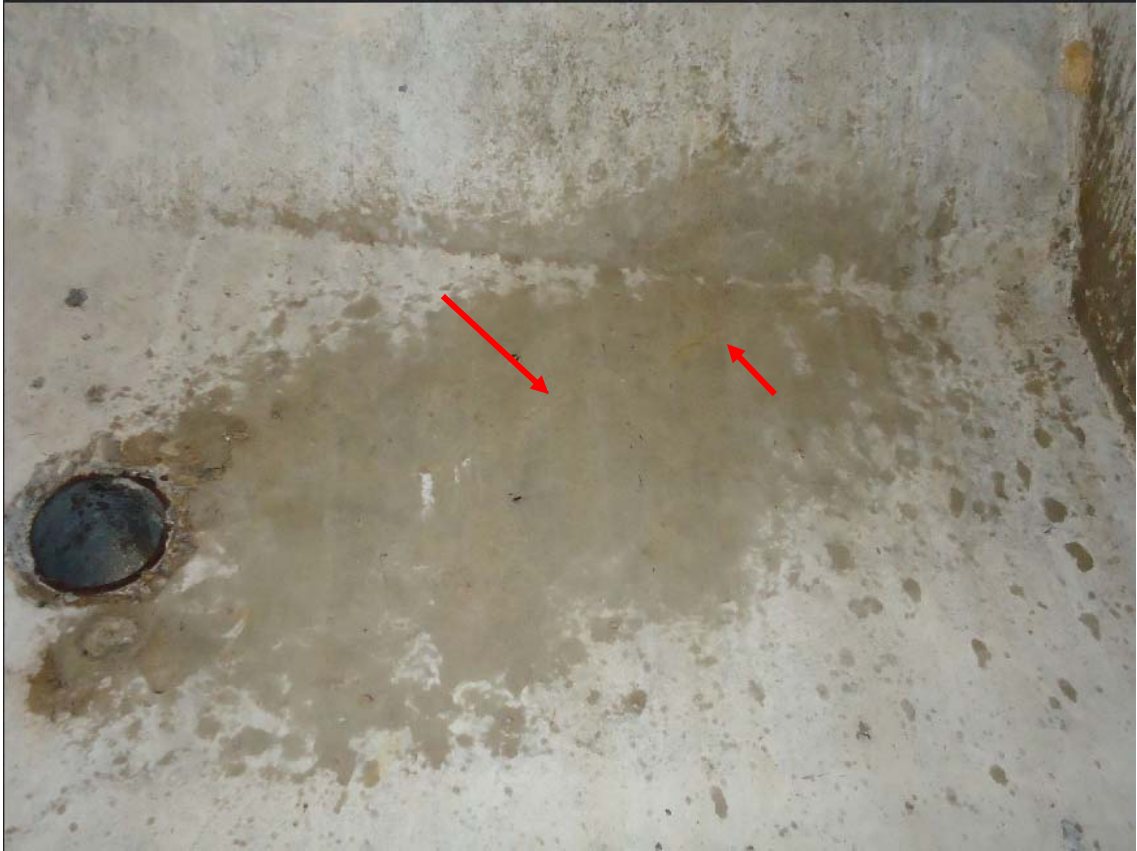
Figure 128. Diagonal cracks from top flange/web interface towards pipe on interior beam (5W-N)
