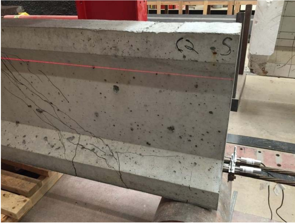
Figure 55. Cracking of C2S
