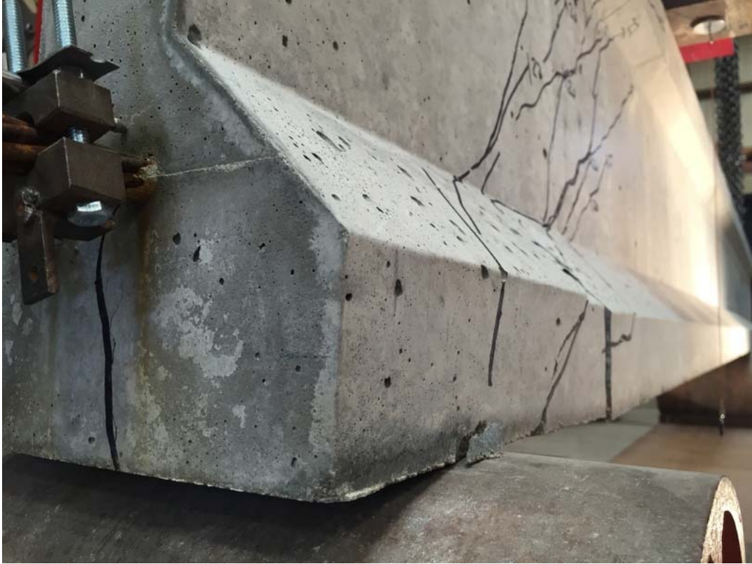
Figure 67. Visual map of cracking of C3S
