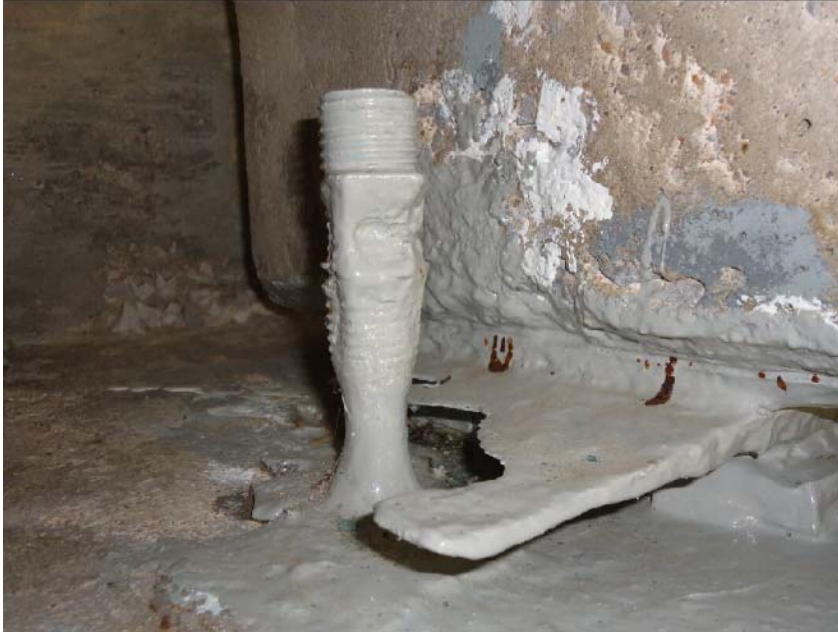
Figure 182. Anchor bolt and bearing plate coated (1S-E)
