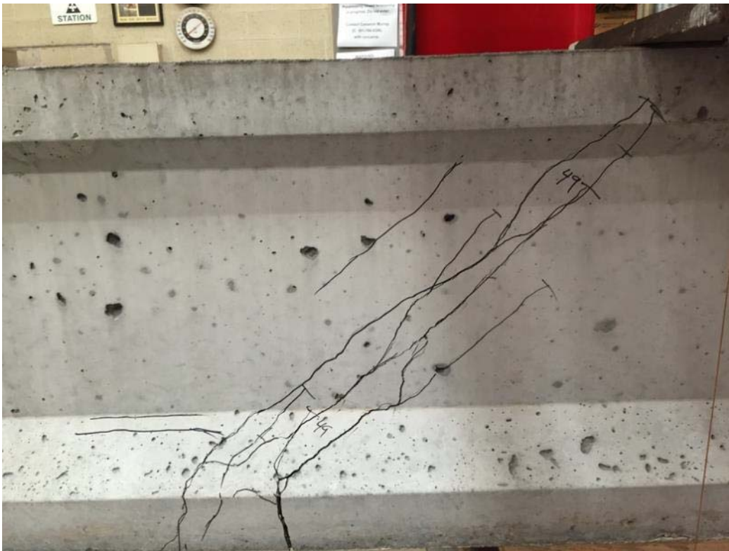
Figure 56. Cracking of C2S
