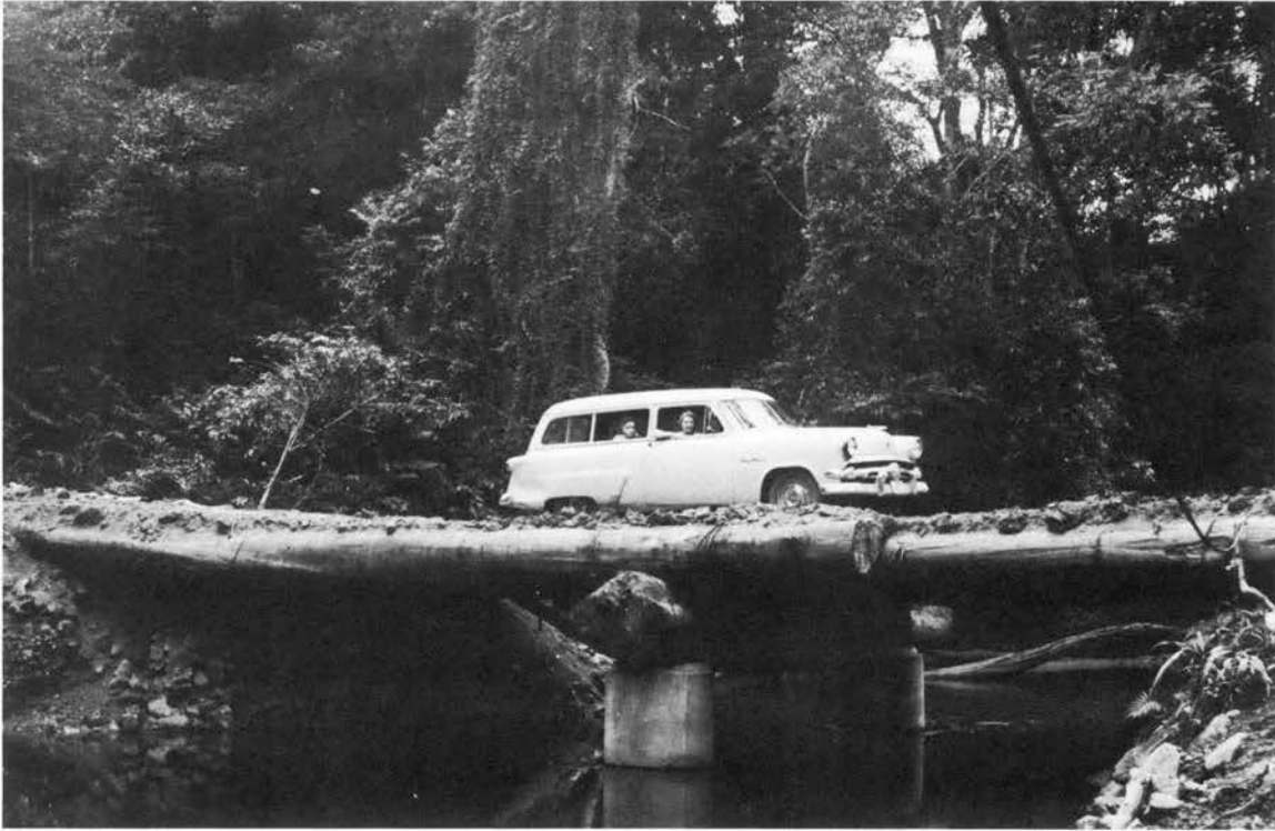
Figure 26. Temporary Bridge on Road Contract
