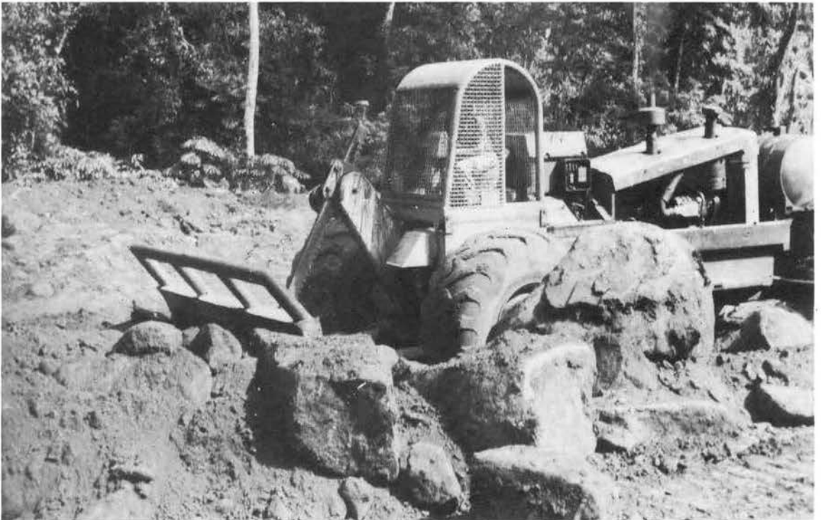
Figure 23. Electric Drive Tractor Moves Boulders for Road Building
