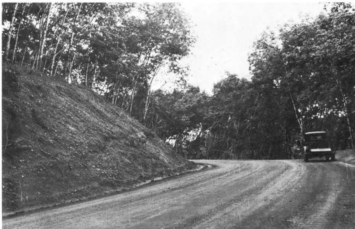
Figure 25. Partially Finished Portion of Road Contract
