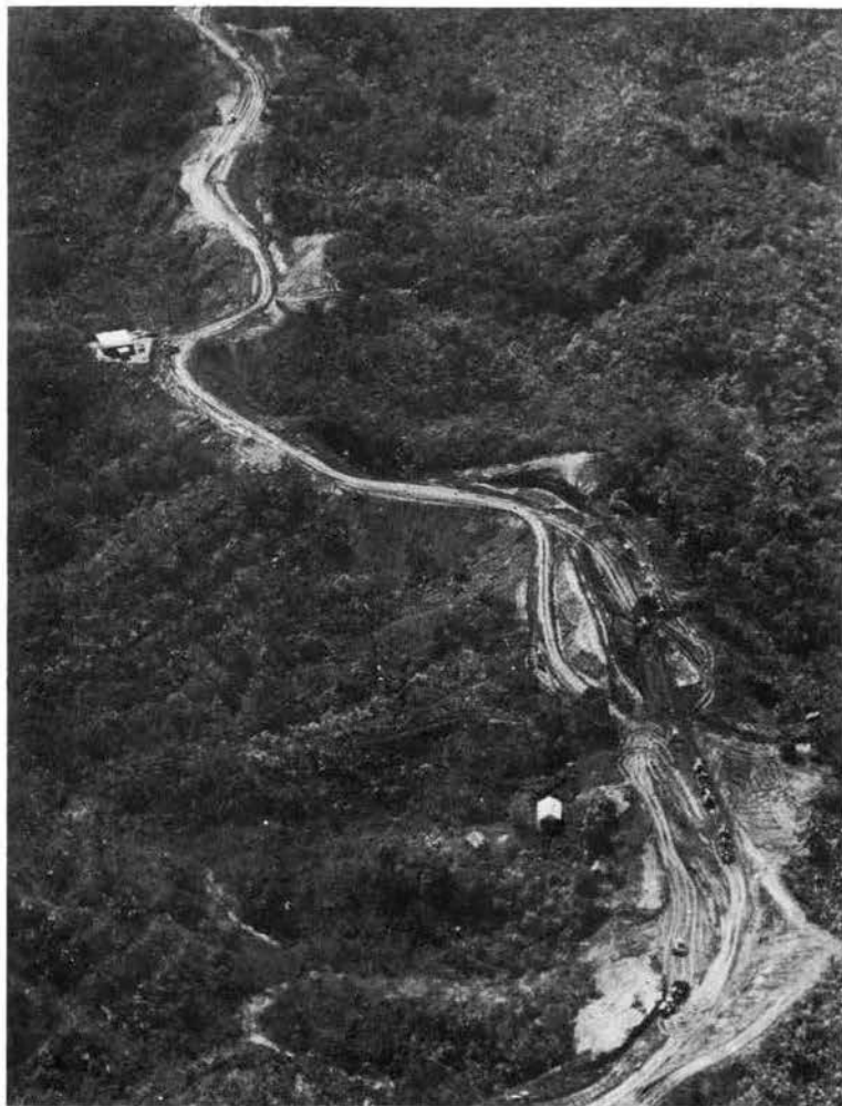
Figure 46. Aerial View of Road Construction and Dense Amazon Jungle
