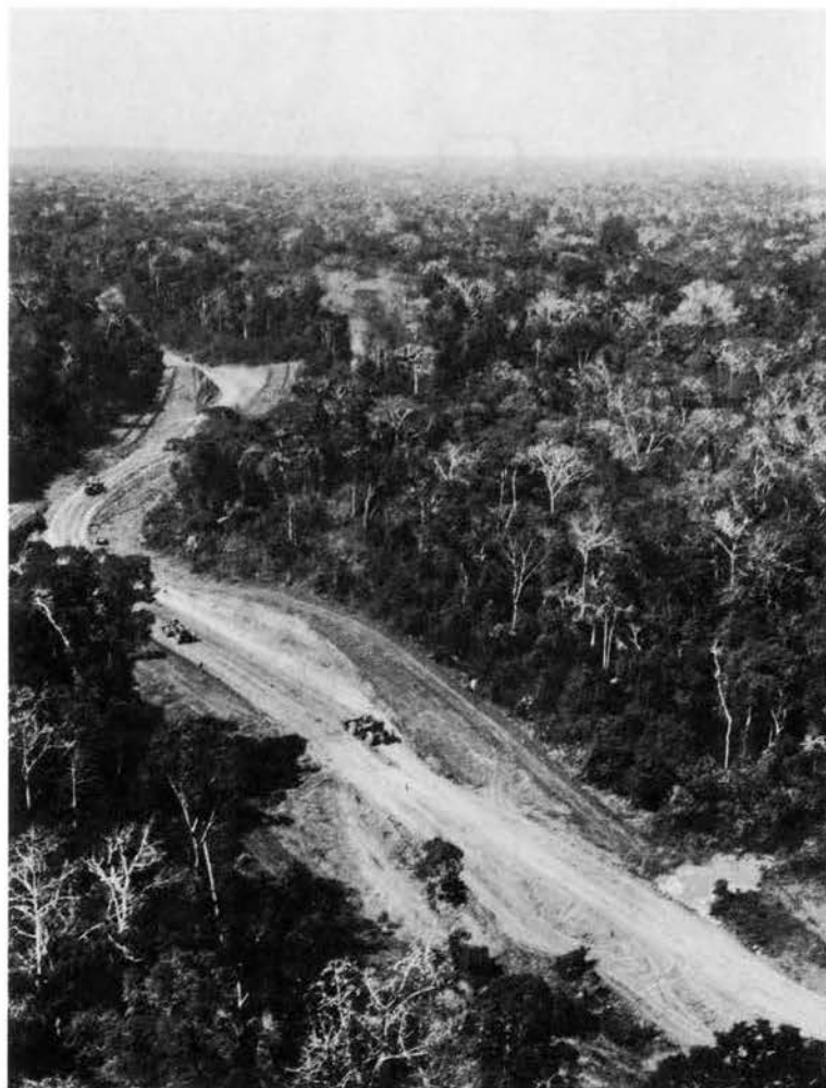
Figure 47. Aerial View of Road Construction and Dense Amazon Jungle
