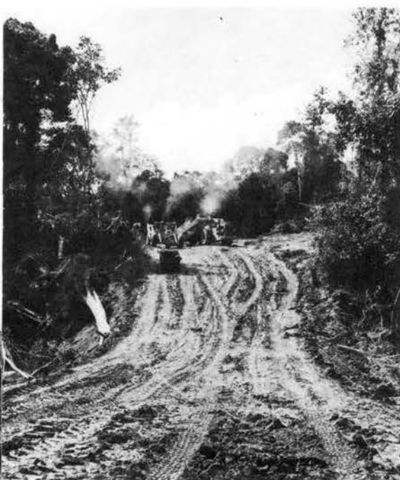
Figure 42. Opening up a "cut" on the LeTourneau Road in Peru
