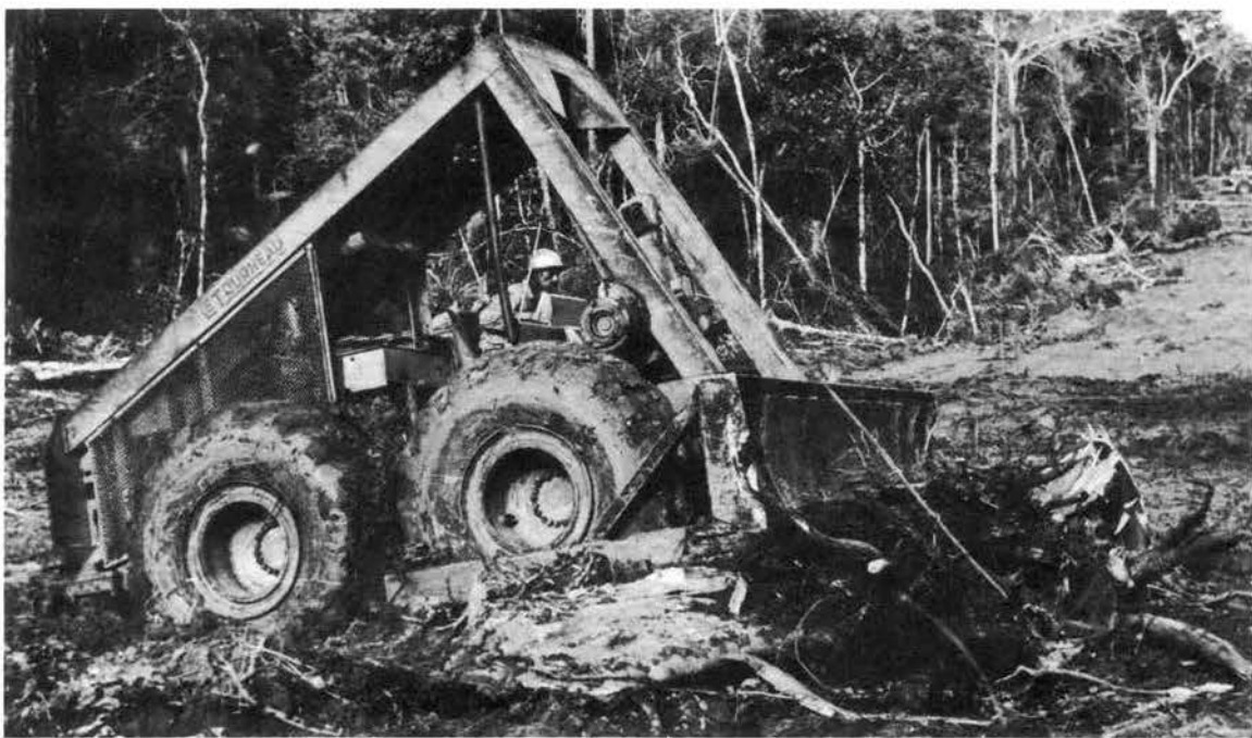
Figure 43. Rubber-tired Bulldozer Clears Right-of-way for Road
