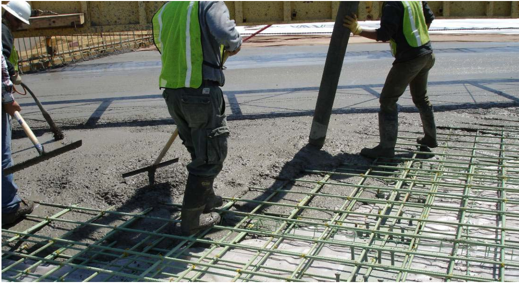
Figure 6. 15 – The Pump Truck Being Used in Construction of Span 2
