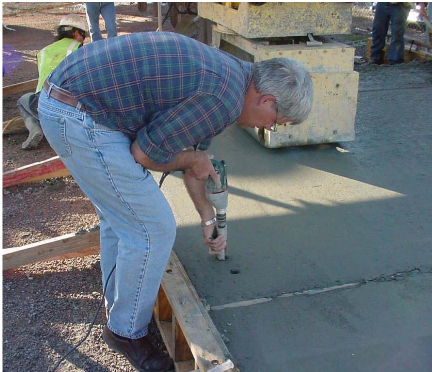
Figure 6.12 – AVA Sampling from the Test Slab
