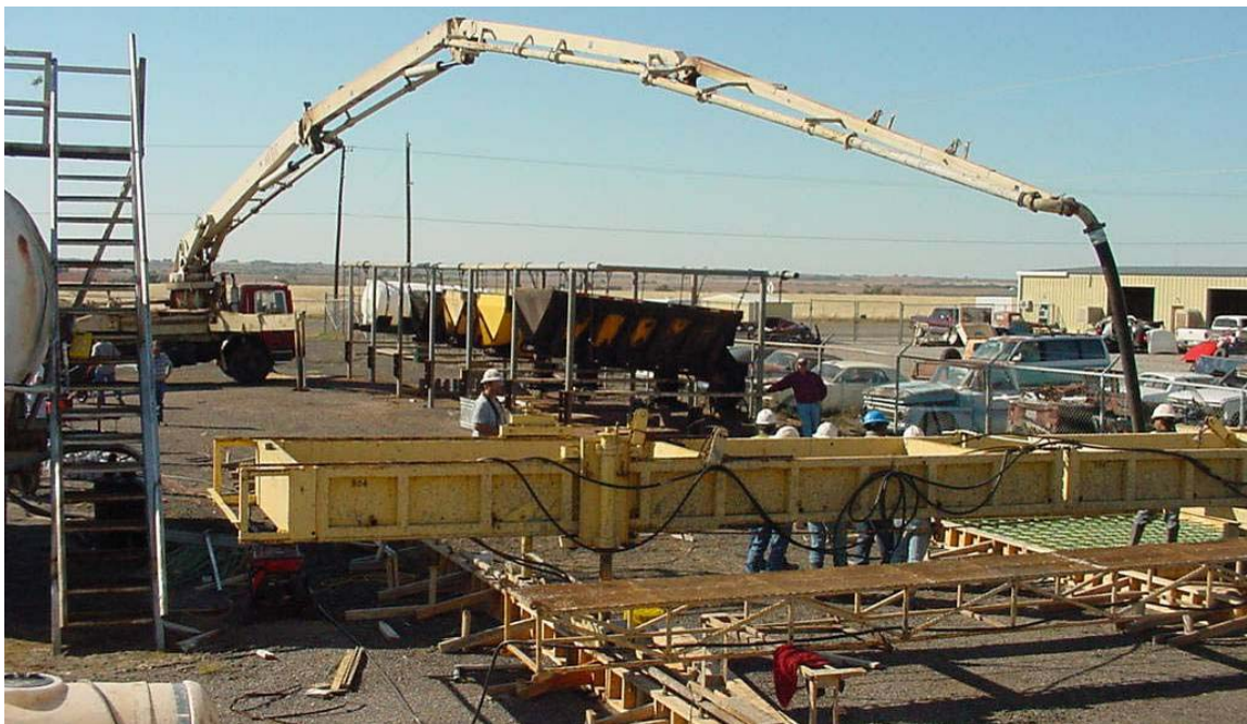
Figure 6.7 – Pump Truck Applying the Cement + Fly Ash Mixture to Test Slab 1
