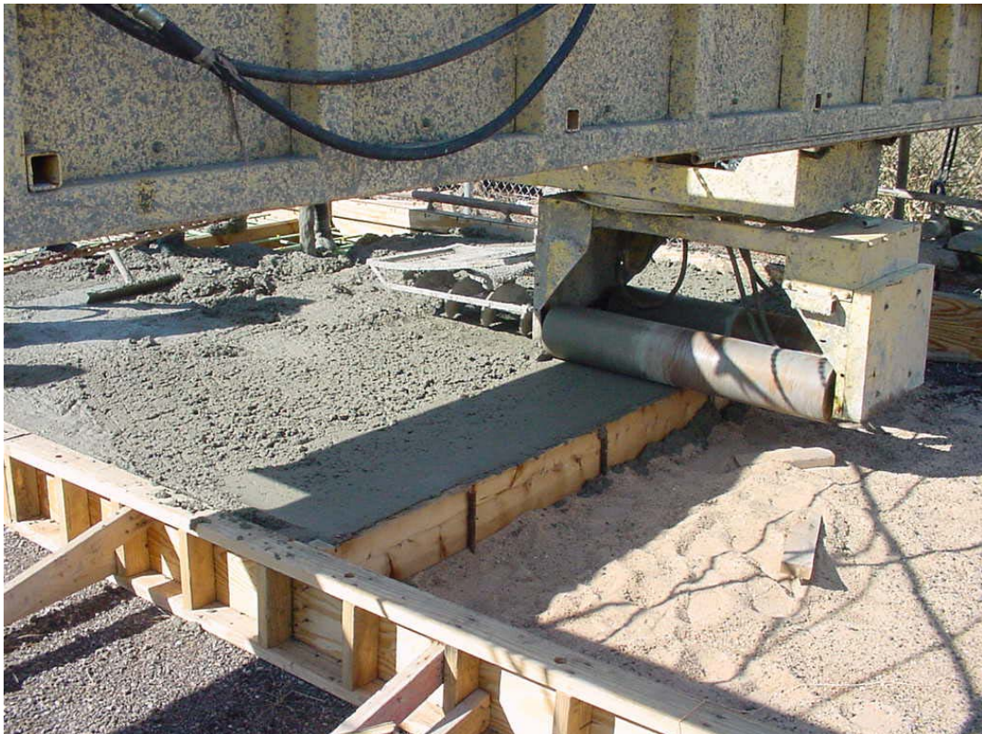
Figure 6. 2 – Mechanical Finisher Used at the Test Slabs
