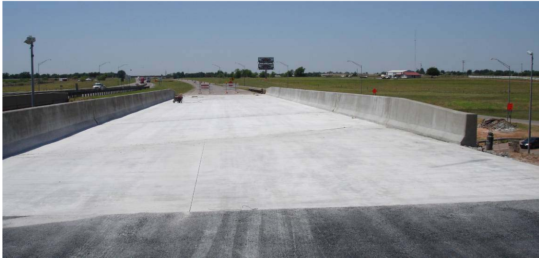
Figure 6. 19– Phase I Bridge Deck after Construction
