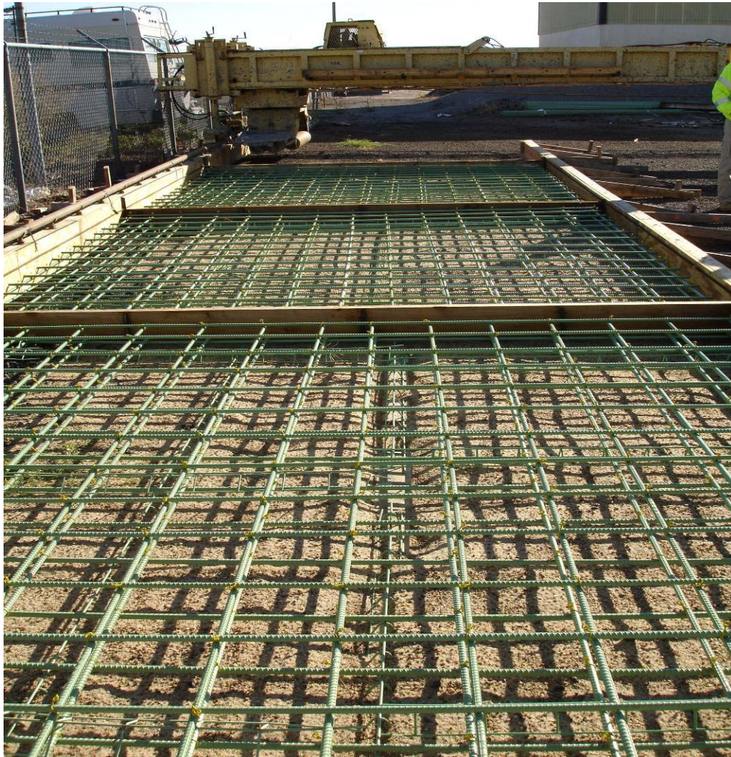
Figure 6. 1 – Formwork and Reinforcing of the Test Slabs
