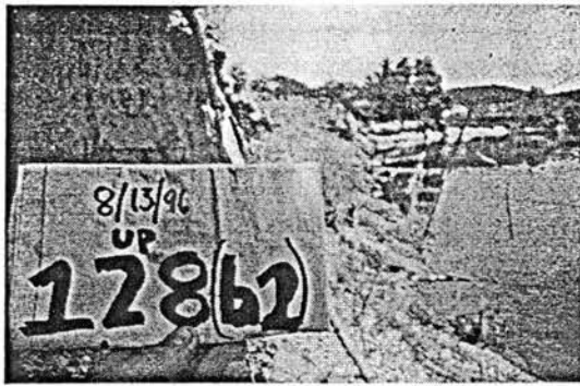
Site 128b2 - upstream view from cross section
