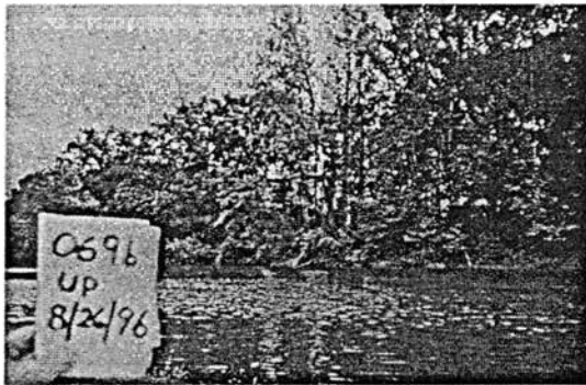
Site 069b - upstream view from cross section
