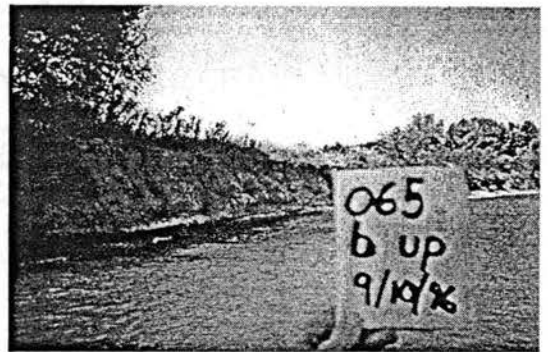
Site 065b - upstream view from cross section
