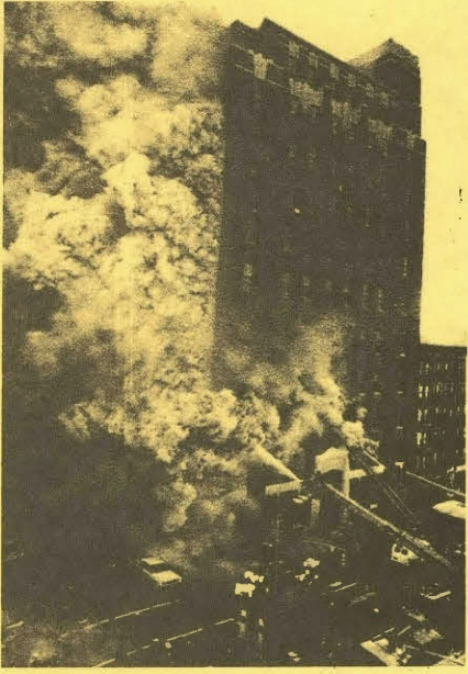
FIRE HITS TELEPHONE BUILDING—Smoke almost envelops a five-alarm fire in a New York Telephone Co. building in lower Manhattan Thursday which injured more than 60 firemen and civilians. The fire knocked out service on police emergency lines and on nearly 200,000 private telephones. (AP)
