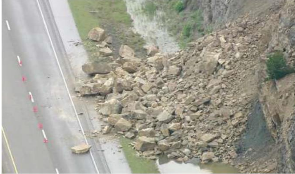
Figure 3. Rockslide on I-35 near Davis, Oklahoma (Source: News Channel 4, KFORD.com)
