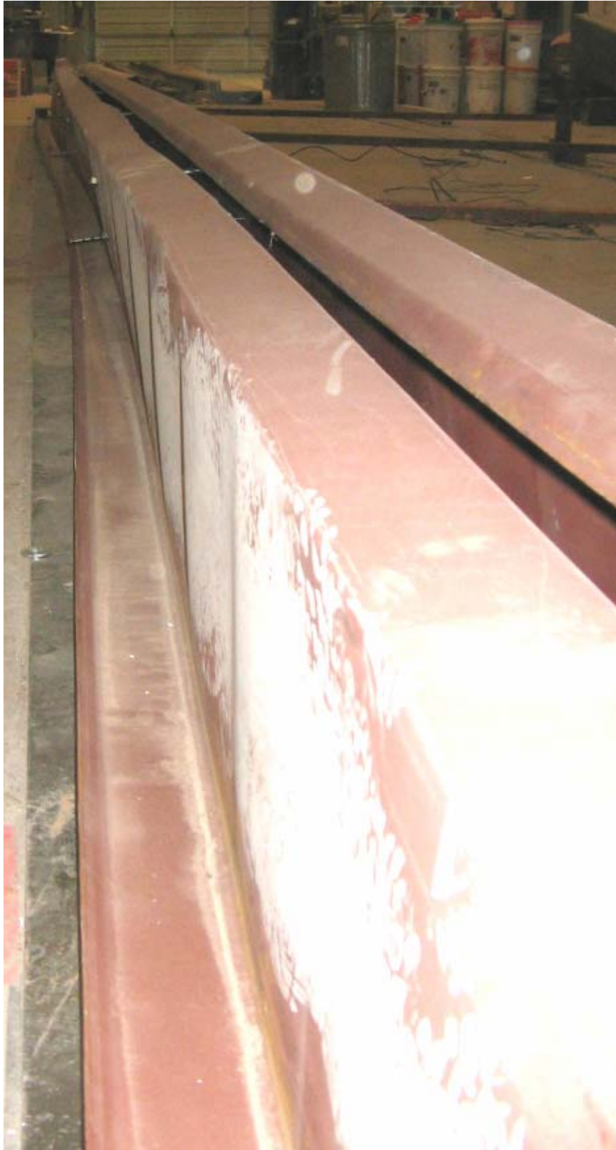
Figure 5.7 Distortional and Local failure for restrained test of purlins with no roof panel
