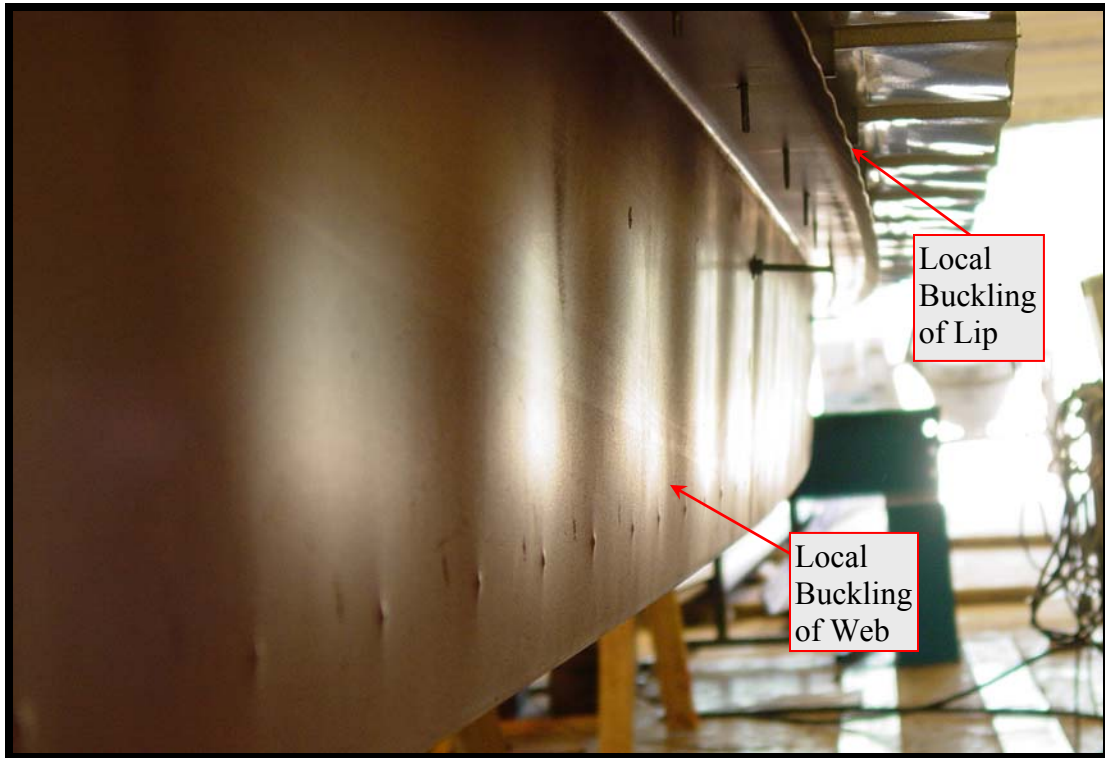
Figure 5.2 Purlins Undergoing Large Side Sway
