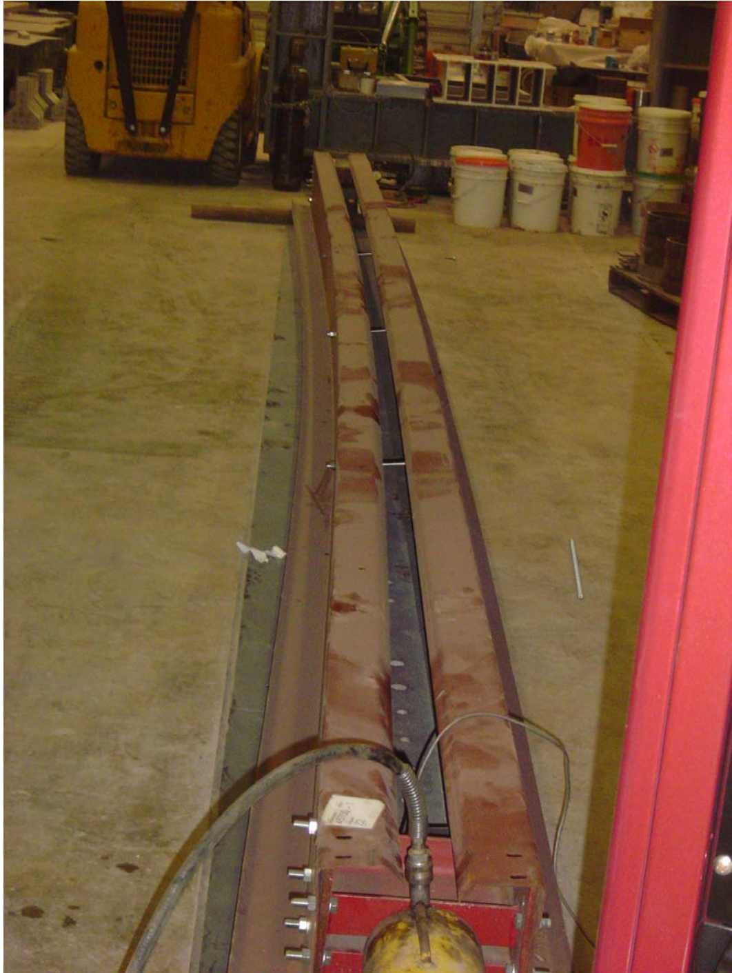
Figure 5.5 Global failure of unrestrained test of purlins with no roof panel
