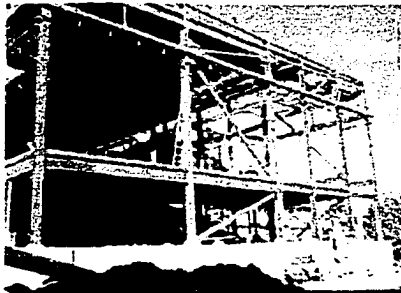
Fig. 2 Steel structure (University of Oklahoma, Norman, OK)
