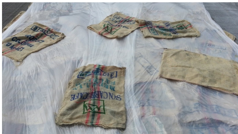
Figure 25 - Wet curing for five days under white plastic sheets
