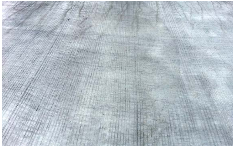
Figure 24 - PAMS curing compound applied by the research team
