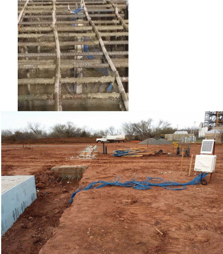
Figure 2.7. Thermocouple installation and Data Logger position after casting the concrete
