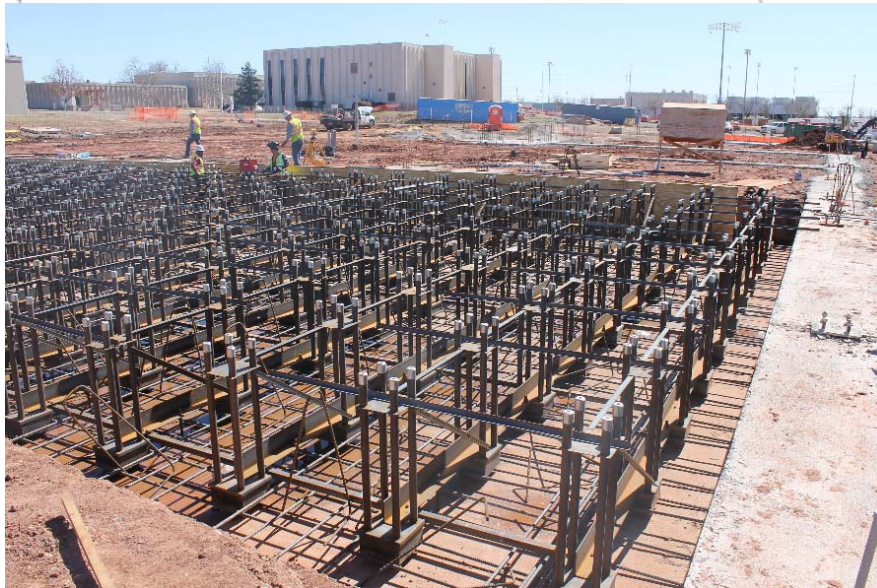
Figure 2.3 – Reinforcing detail in the mass floor
