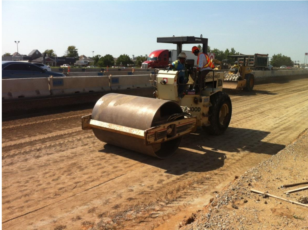
Figure 5.7 ICA compaction procedure in progress.
