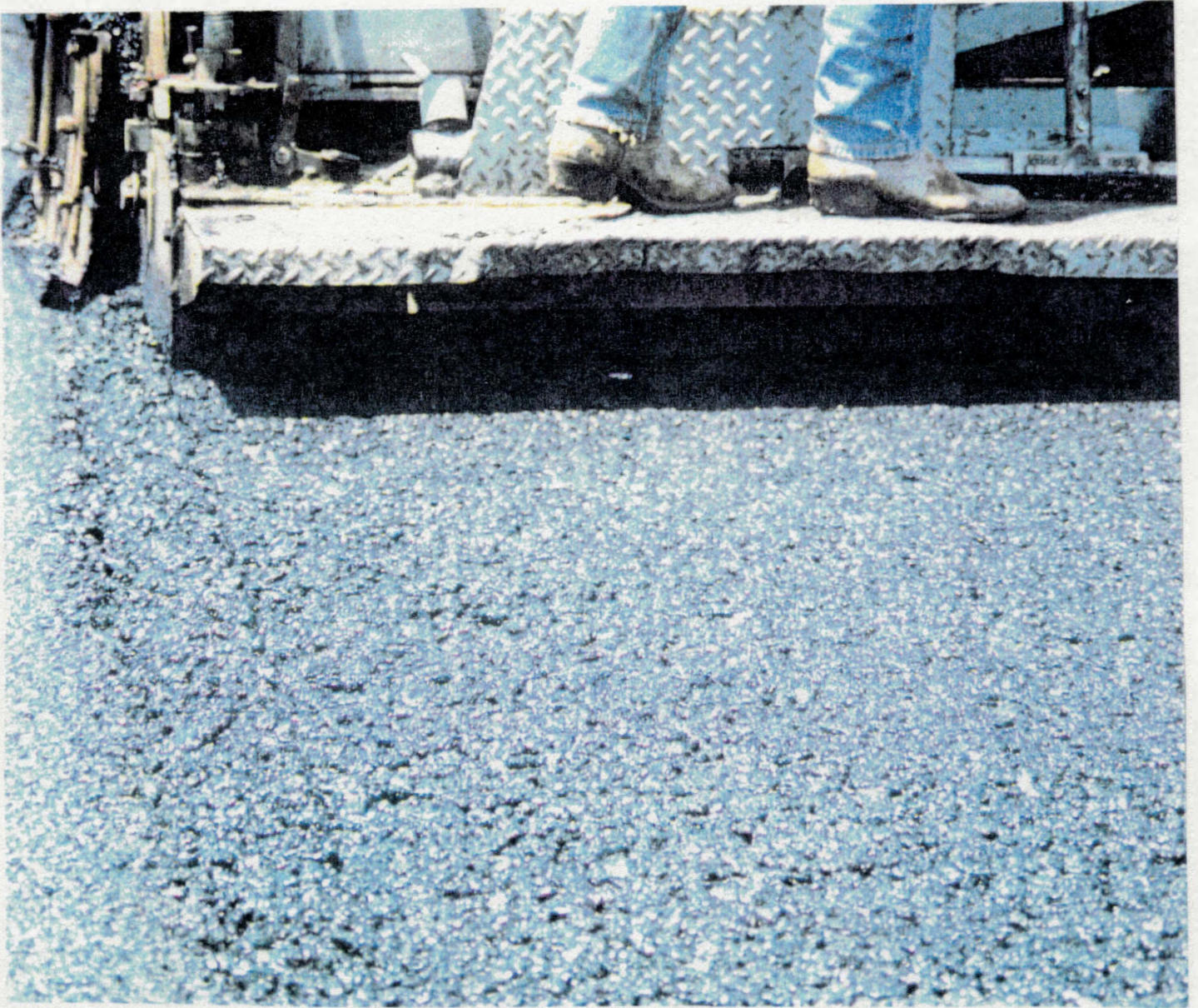
PHOTO 3. LAYDOWN AT SITE 6.
