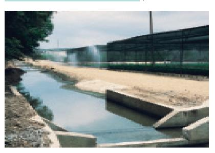
In a capture and recycle system, irrigation runoff from nursery beds and houses in production areas is collected by a system of channels or ditches leading to retention basins.
