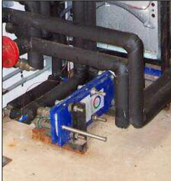
Figure 3.5 Plate heat exchanger.
