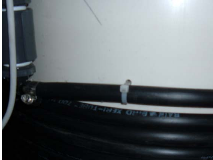
Figure 2: Zip tie attached to irrigation tubing at top of PVC support
