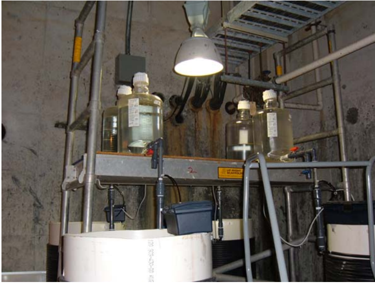
Figure 5: Scaffolding with carboys on top
