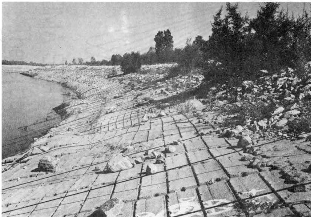
Figure 43. Island 63 Revetted Area Underlain With Filter Cloth
