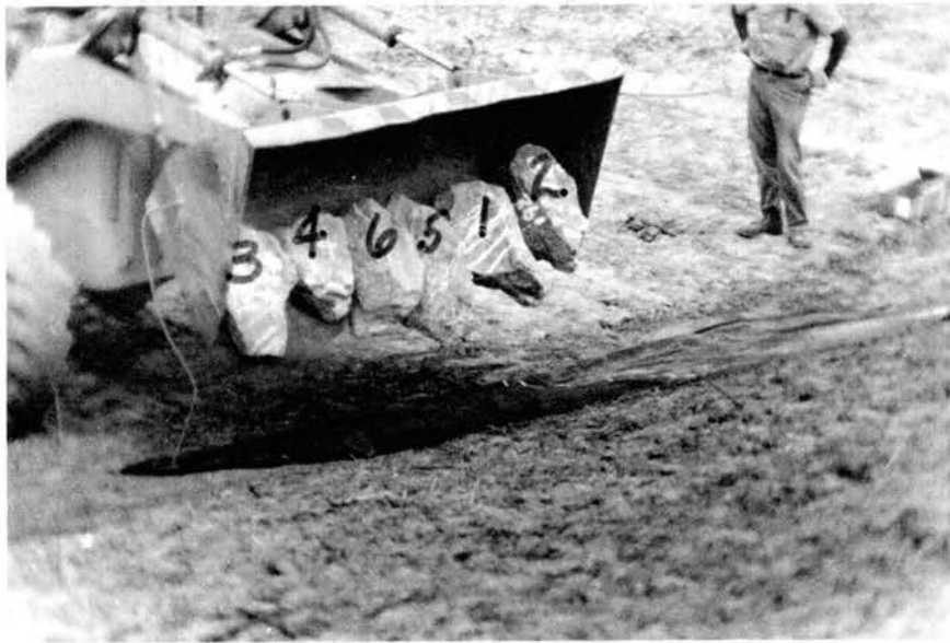
Figure 34. Stones Being Dropped From Bucket
