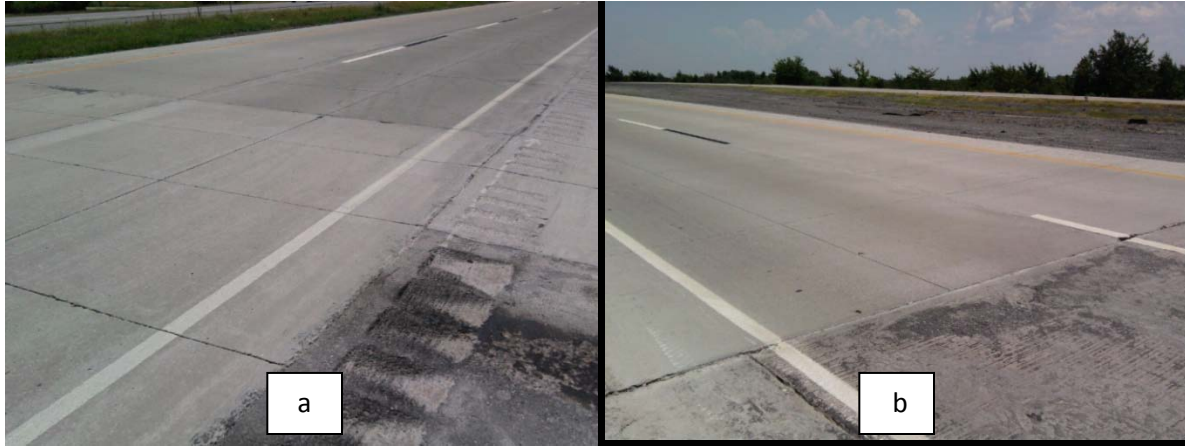
Figure 2.16 - Photo a showing start and photo b showing end of the south bound overlay.
