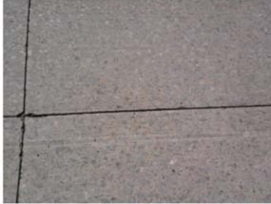
Figure 2.21 – Polishing of the overlay surface.
