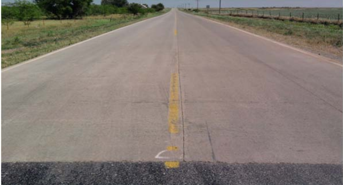
Figure 2.51 - Photo shows the overlay from south direction (looking towards north).
