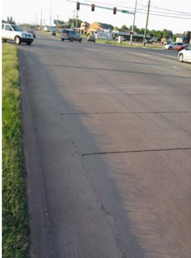
Figure 2.33 - Excellent condition of panels on US 177 from the south.
