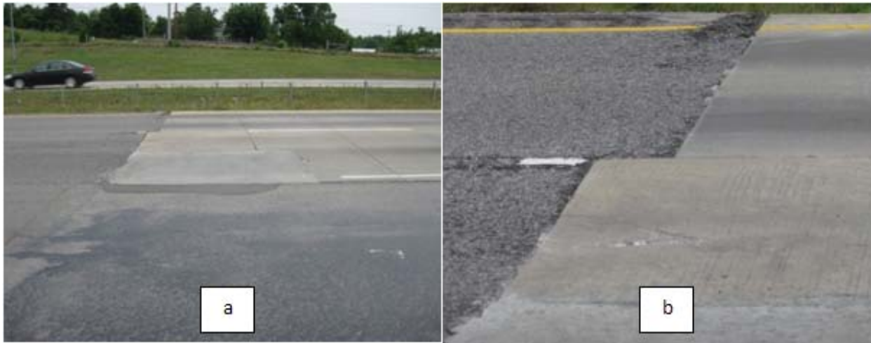
Figure 2.10 - Initial panel replacement at the start of overlay as seen in photo a, and in photo b we see how there is an elevation difference between the leaving asphalt panel and approaching concrete panel.
