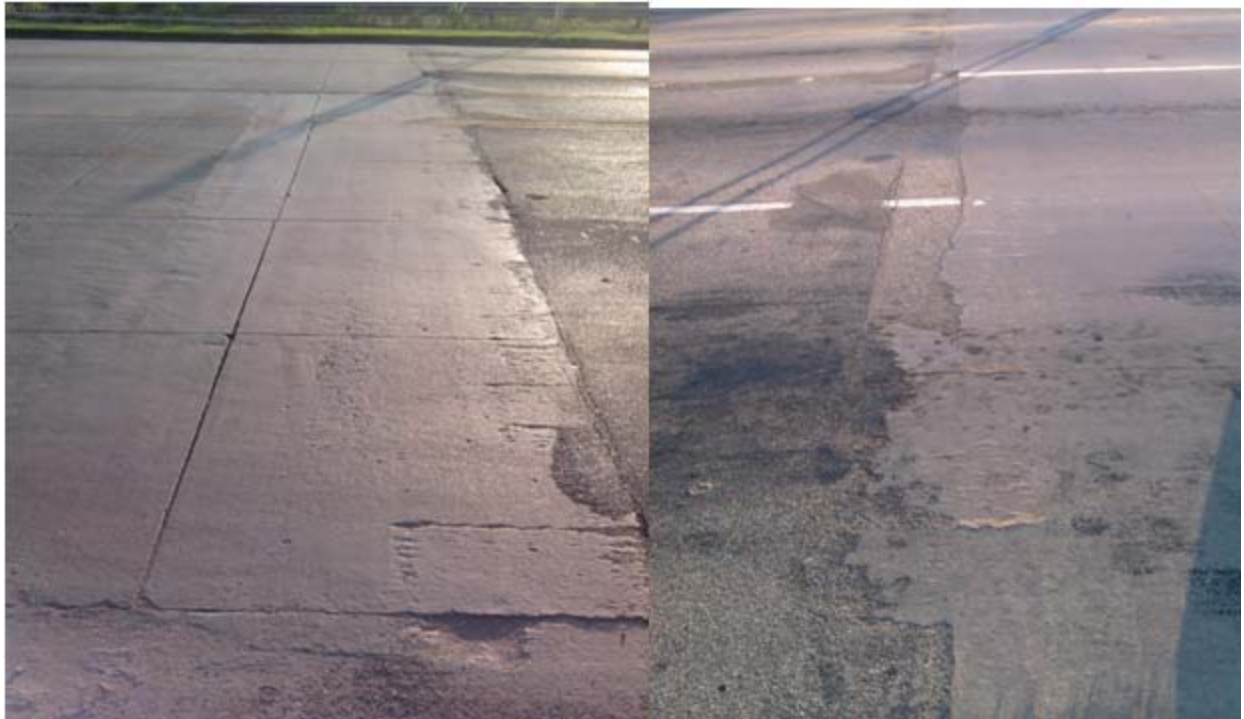
Figure 2.35 - Approach on US 177 from north showing absence in panel failures. Note the small difference in the elevation between the approach and leave pavements.
