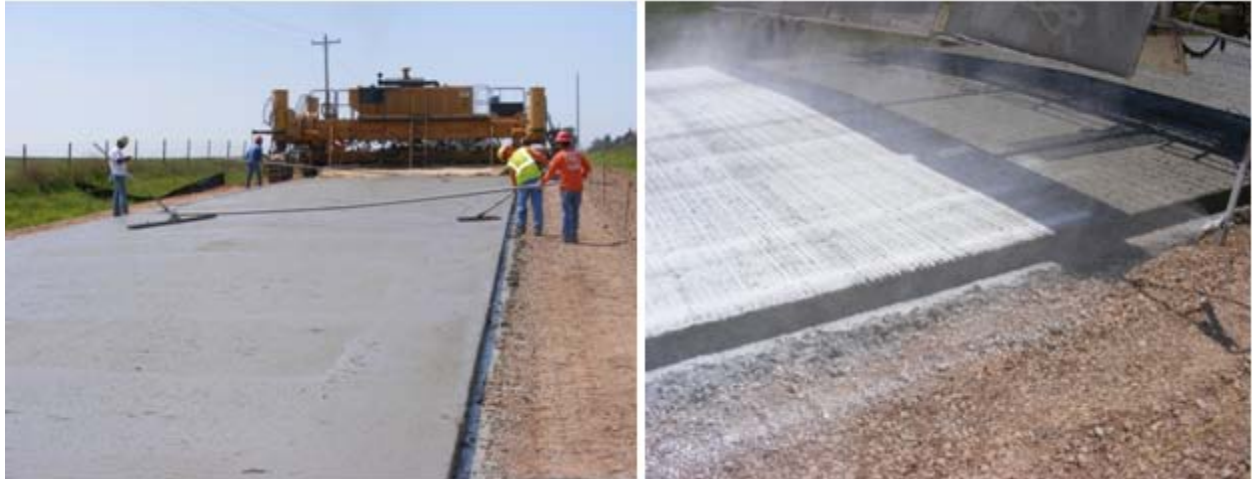
Figure 2.49 - Photos show the construction of the overlay. (Photos in Figs 2.48 & 2.49 courtesy of Chris Westlund, ODOT).
