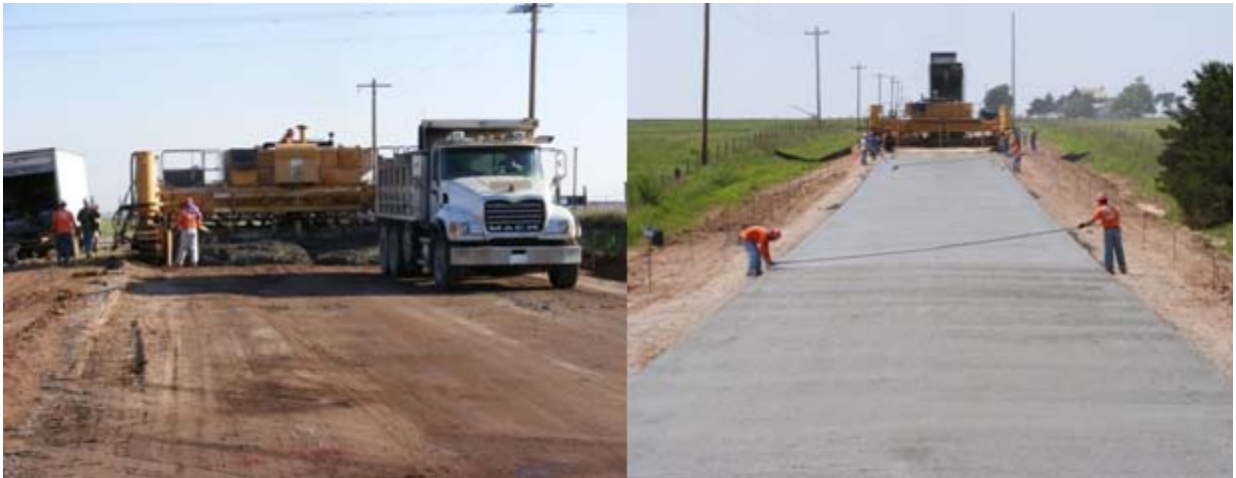
Figure 2.48 - Photos show the construction of the overlay.
