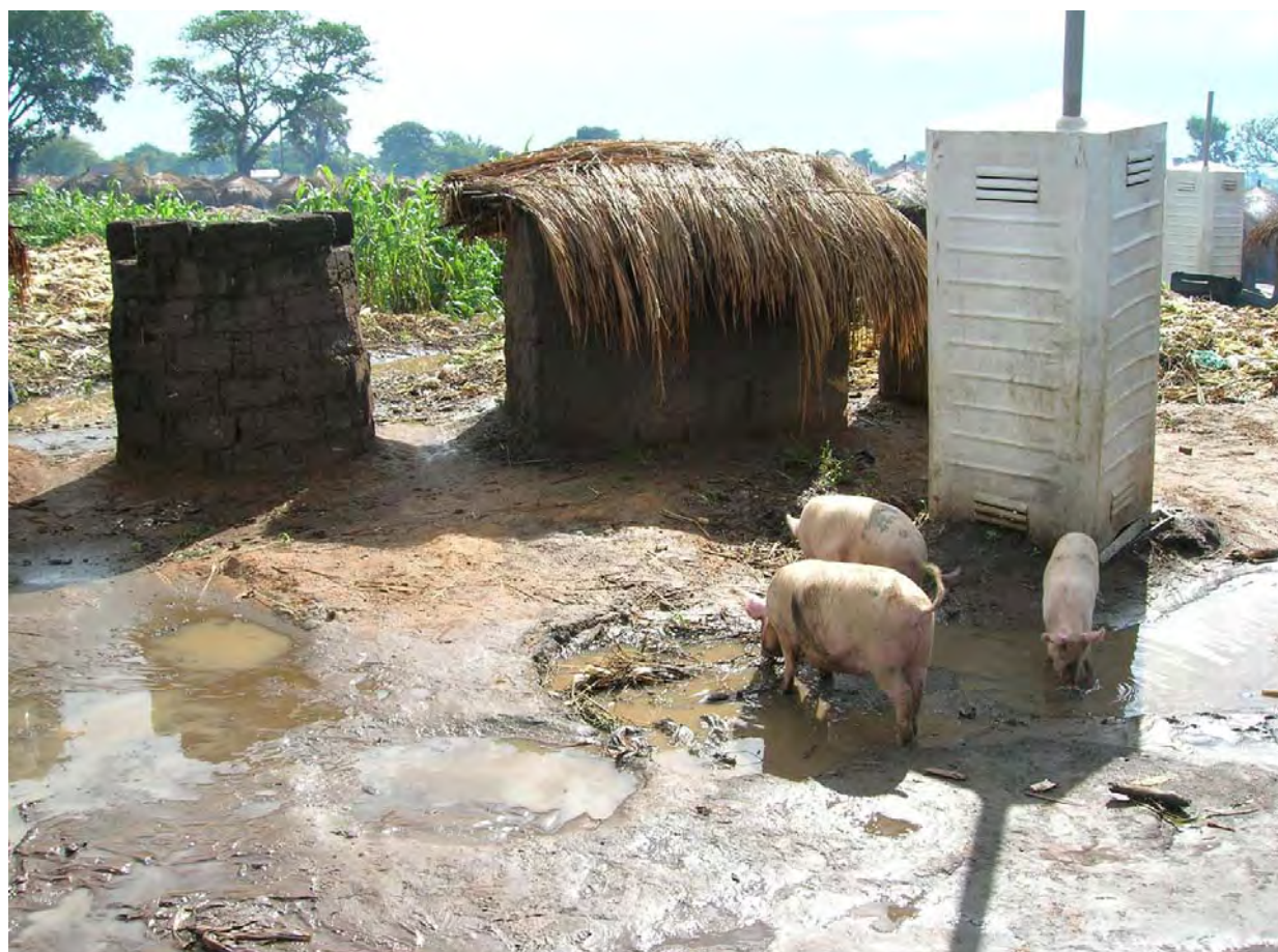
Overflowing pit latrine at Agweng IDP Camp (Photo: Elliott Green)
