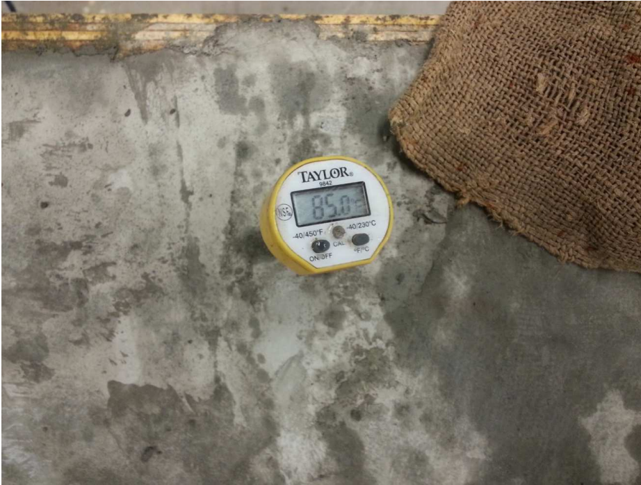
Figure 17 Thermometers were also embedded in concrete to take immediate readings
