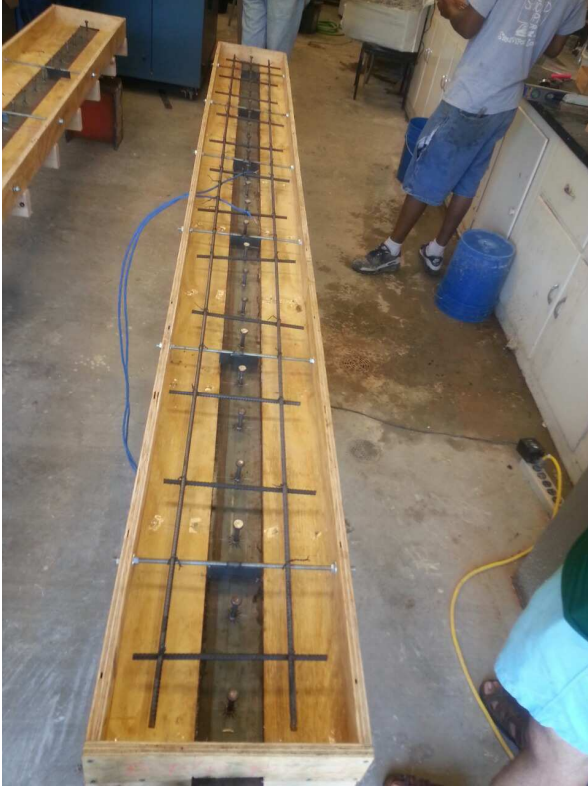
Figure 15 Thermocouples embedded in concrete deck slab
