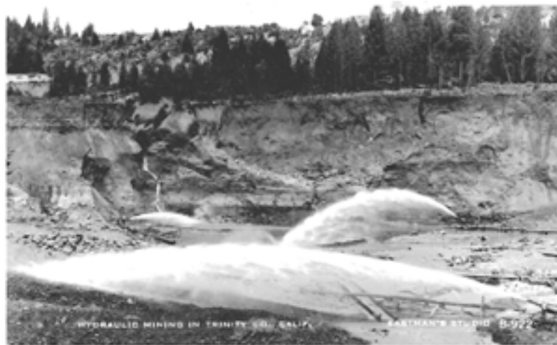
Industrial hydraulic mining scene in the Trinity River Basin ca. 1940. The location of this mine is unknown, but note the hydraulic “Giants” operated by a single individual with a counterweight. Note that the working face has been caved-down and the debris is being pushed towards the sluice. Eastman photo postcard. Ca. 1940s. Authors’ personal collection.
