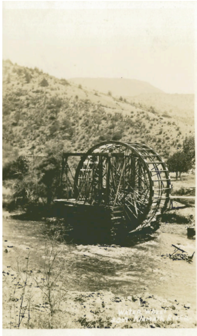
Waterwheel. Photo ca. 1910. This waterwheel is of the typical design used in early placer mining on the Trinity River. This wheel was located on the upper-Klamath River. Photo postcard. Authors' personal collection.
