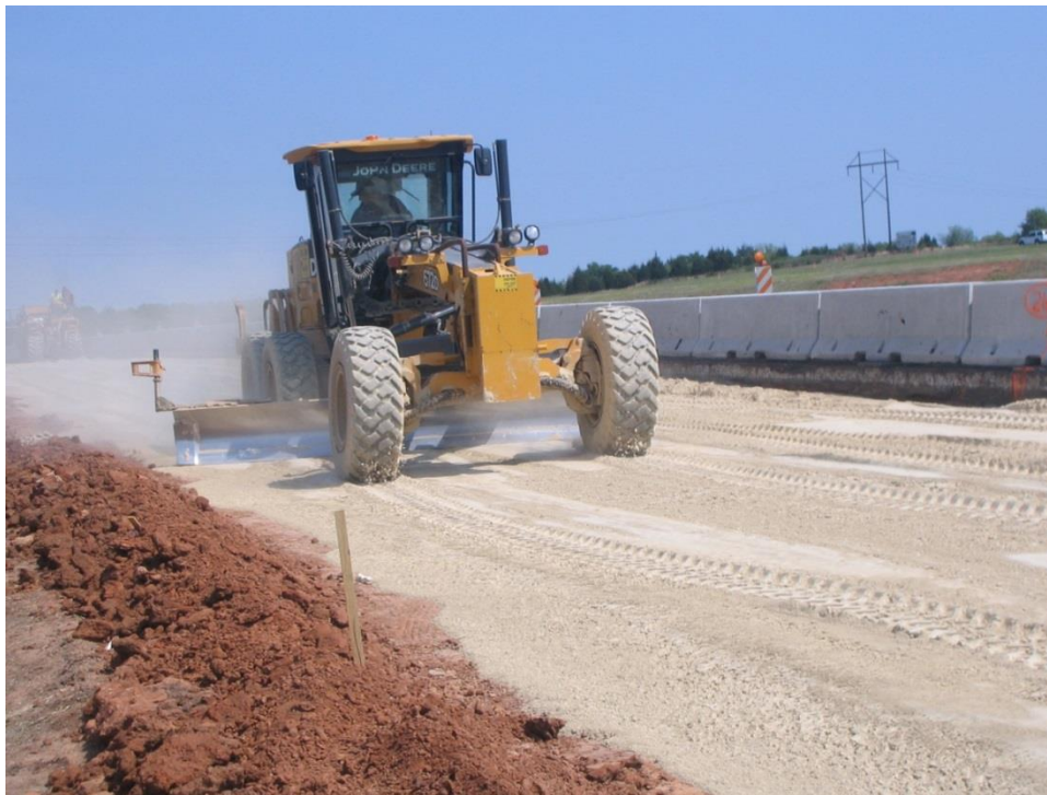
Figure 3-53 A Motor Grader Spreading CFA
