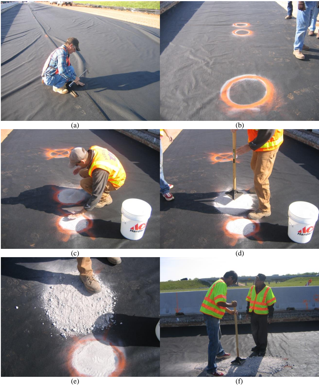
Figure 3-63 Hand Placement of Aggregate Base Material
