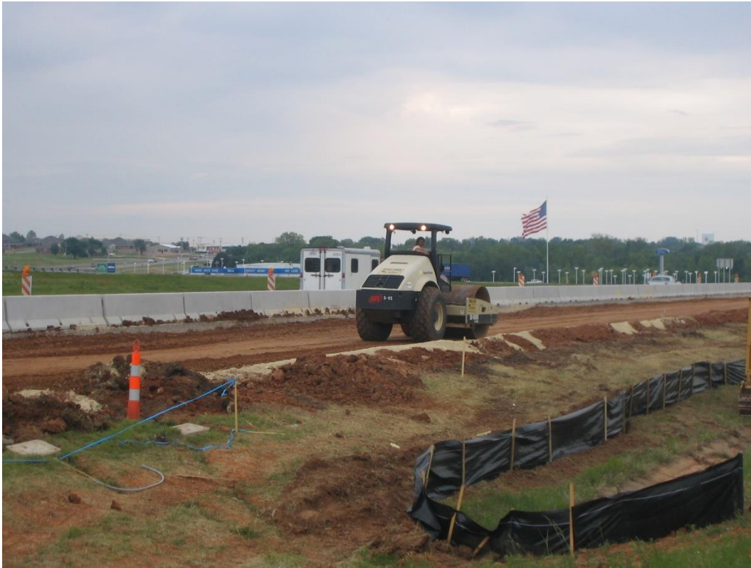
Figure 3-59 Compaction of Stabilized Subgrade Layer
