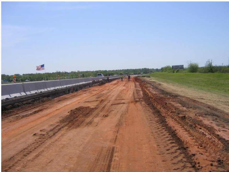
Figure 3-2 Instrumentation Site Before Construction, Looking South
