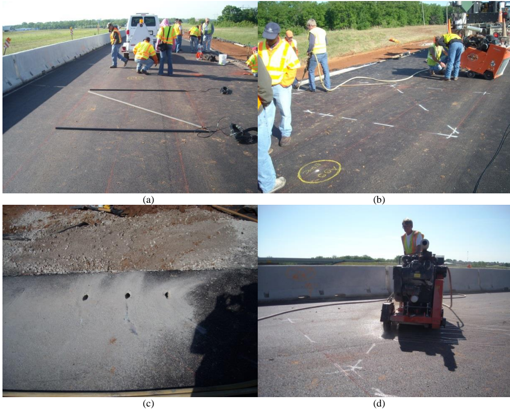
Figure 3-70 Installation of Dynax ® Axle Sensors
