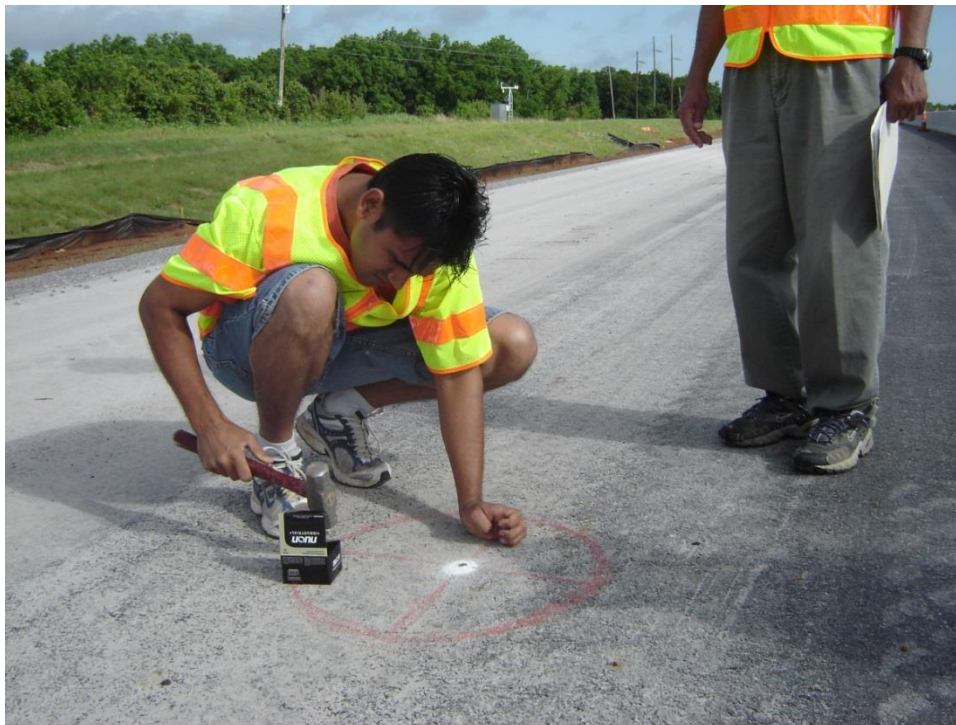
Figure 3-78 Driving Nails on the Identified Stations
