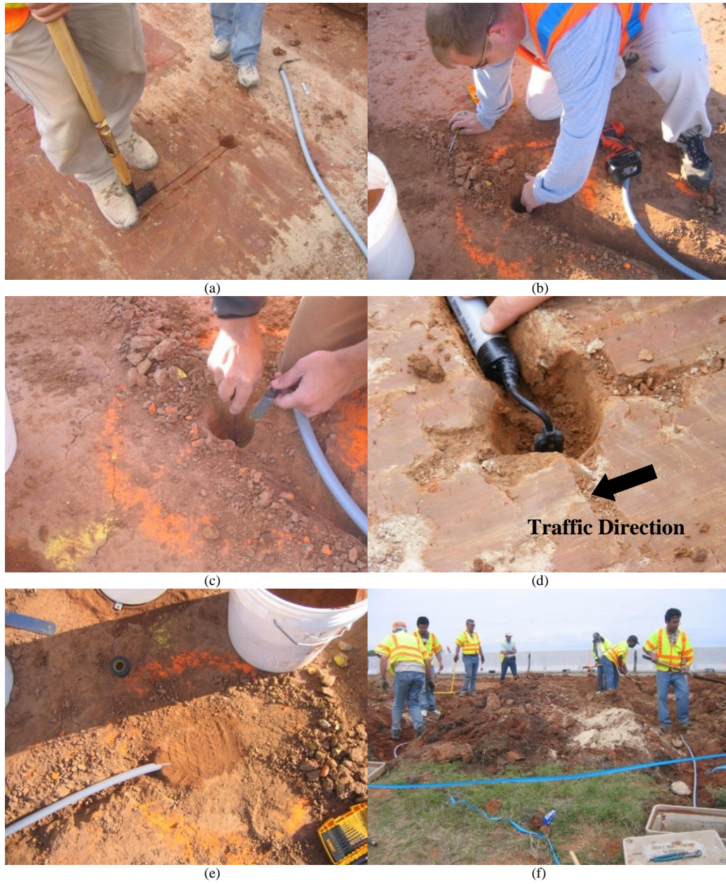
Figure 3-58 Installation of Moisture Probe on Subgrade
