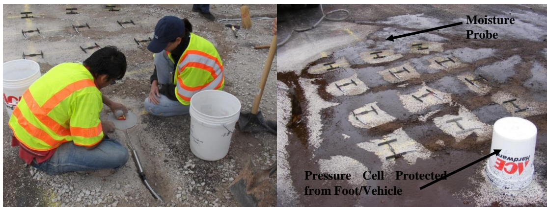
Figure 3-67 Installation of Earth Pressure Cell and Moisture Probe
