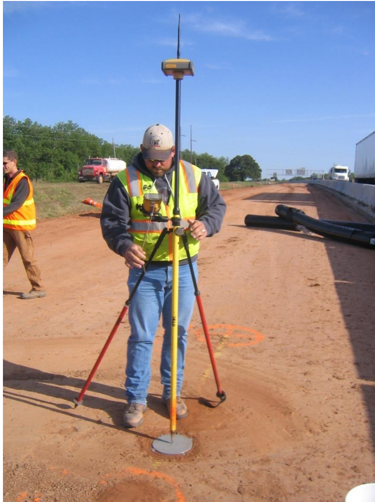
Figure 3-61 Marking Location of Earth Pressure Cell using GPS
