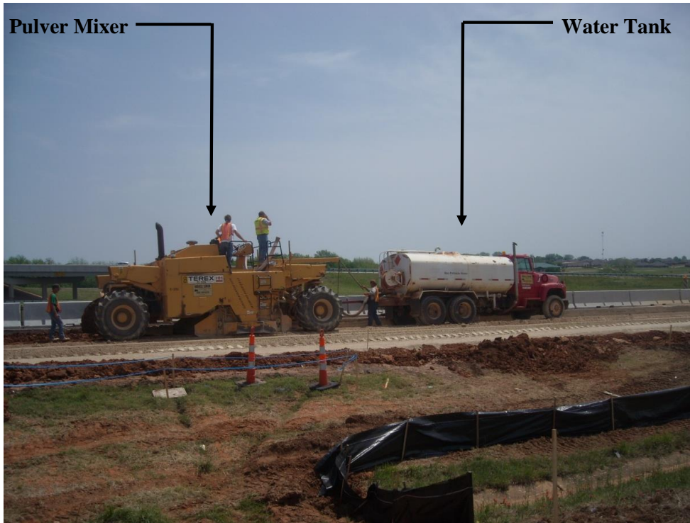
Figure 3-54 Water Tanker and Pulver Mixer Working at the Site
