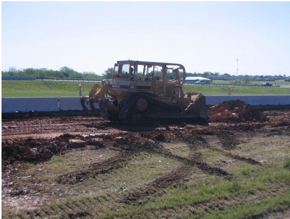
Figure 3-49 Grading of Subgrade Soil
