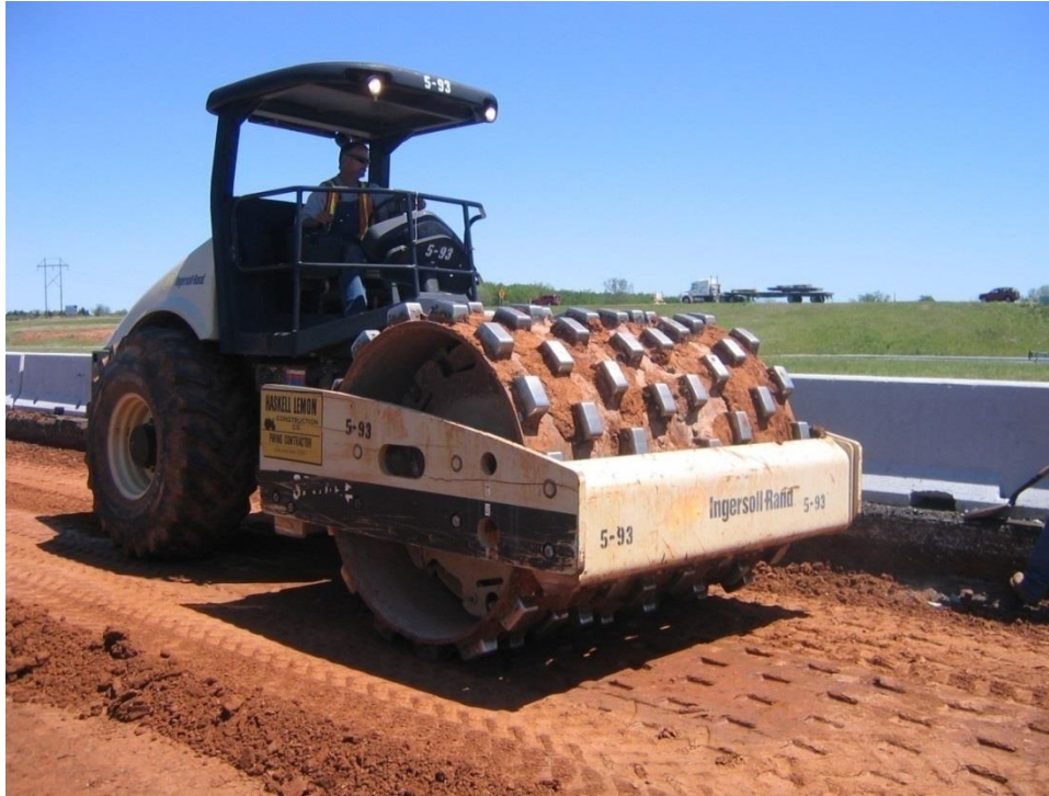
Figure 3-50 Compaction of Subgrade Soil
