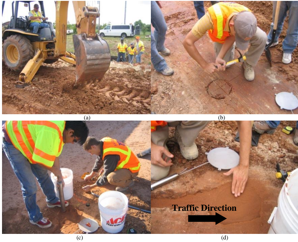
Figure 3-56 Installation of Earth Pressure Cell on Subgrade
