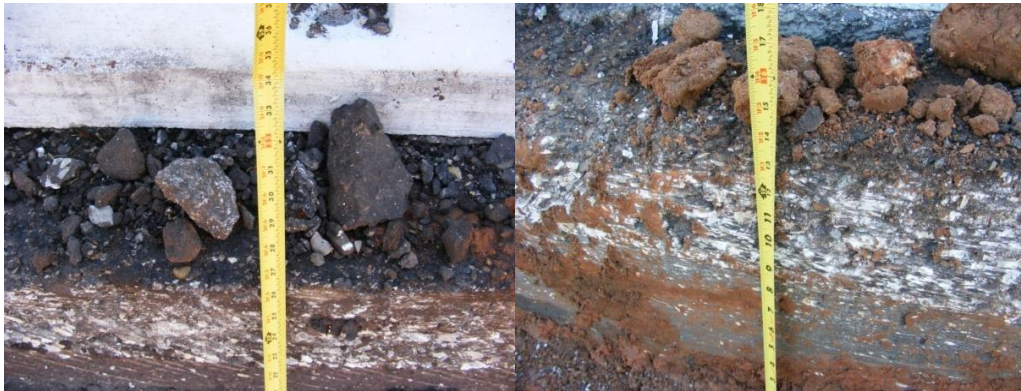
Figure 3-47 After Excavation of Weak Subgrade Soil
