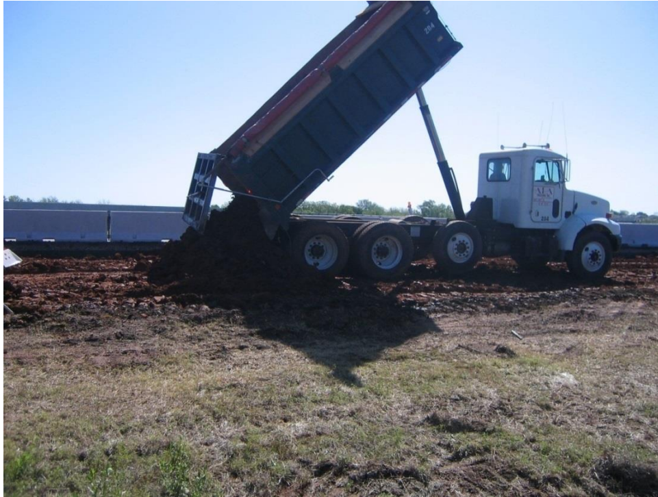
Figure 3-48 Backfilling with Imported Soil
