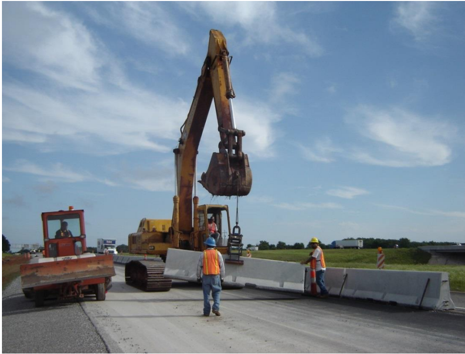
Figure 3-79 Removal of Concrete Barriers
