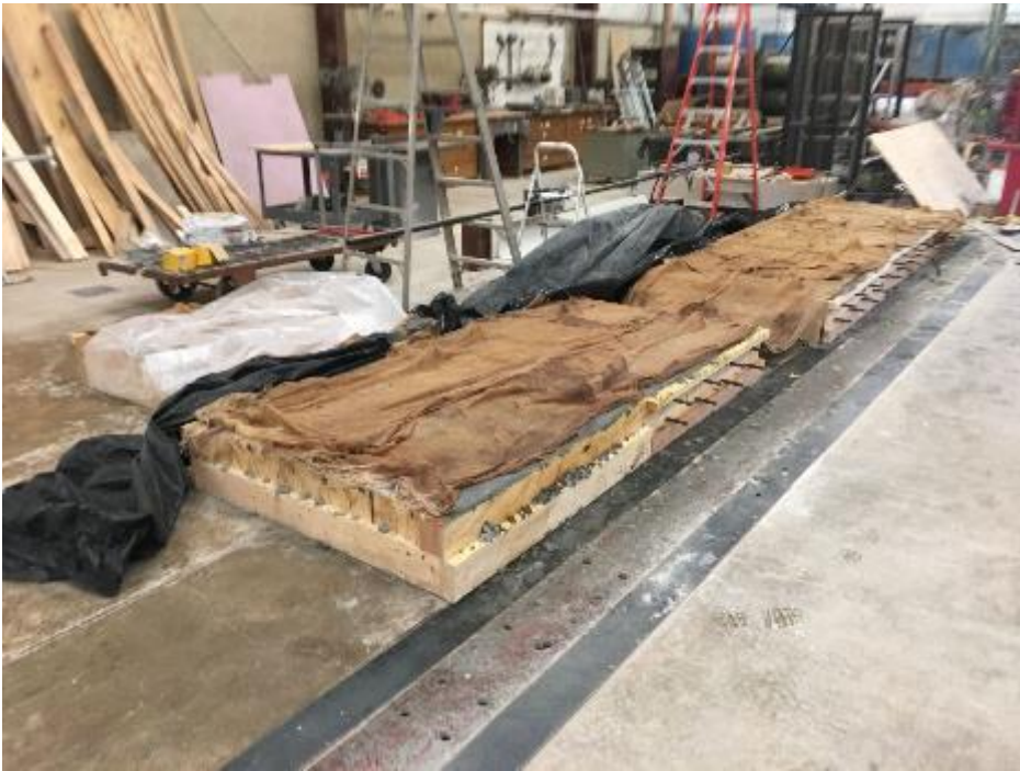
Figure 27. Slab panels curing covered in burlap
