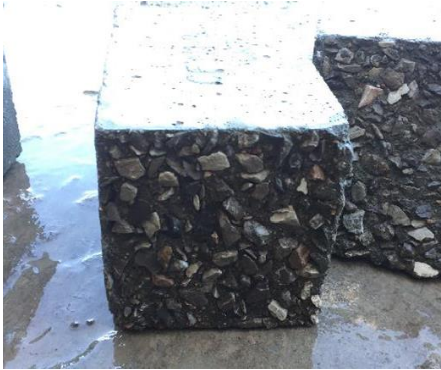
Figure 16. Exposed aggregate surface after power washing
