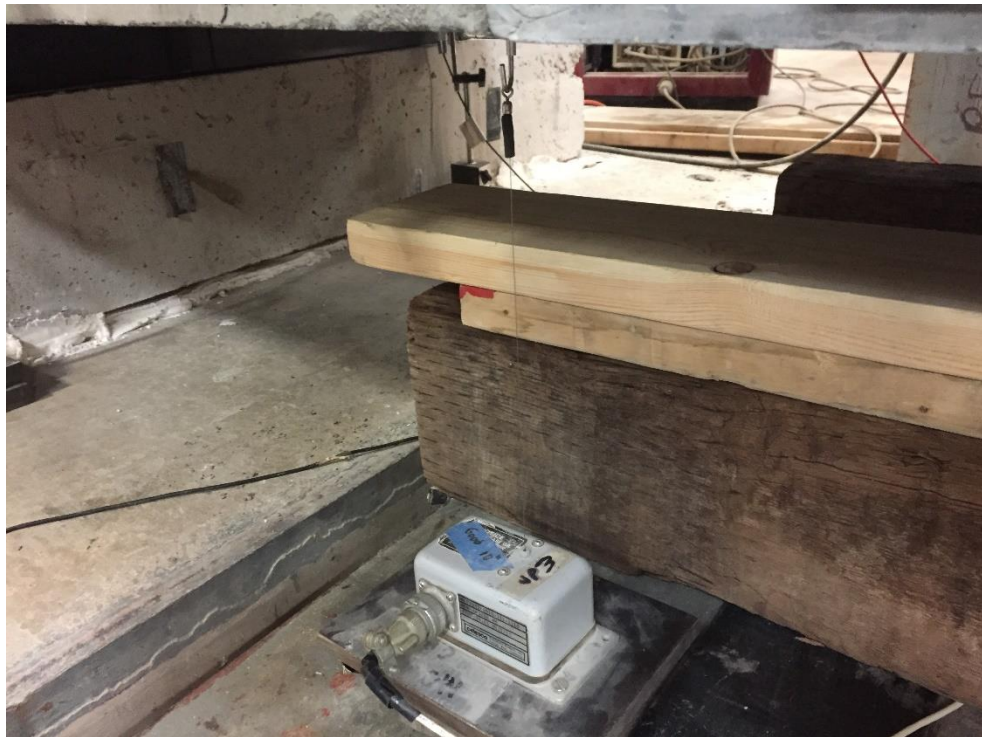
Figure 100. Wire potentiometer attached to underside of slab prior to testing
