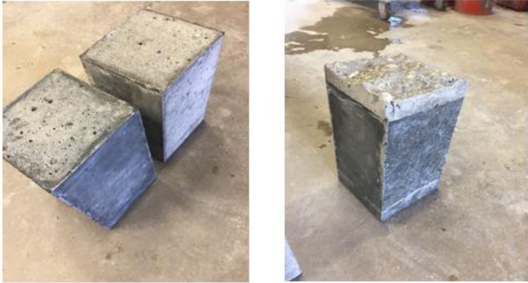
Figure 32. Interface failure (left) and base concrete failure (right)
