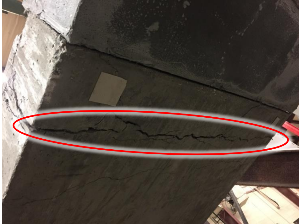
Figure 48. Major cracking underneath load point for slab 2
