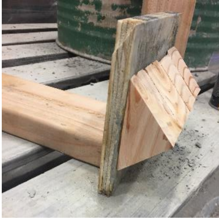
Figure 13. Wood insert for shear key
