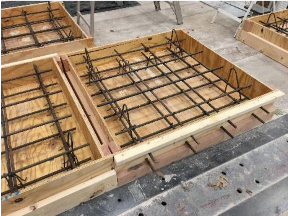
Figure 26. Rebar layout prior to casting slab panels
