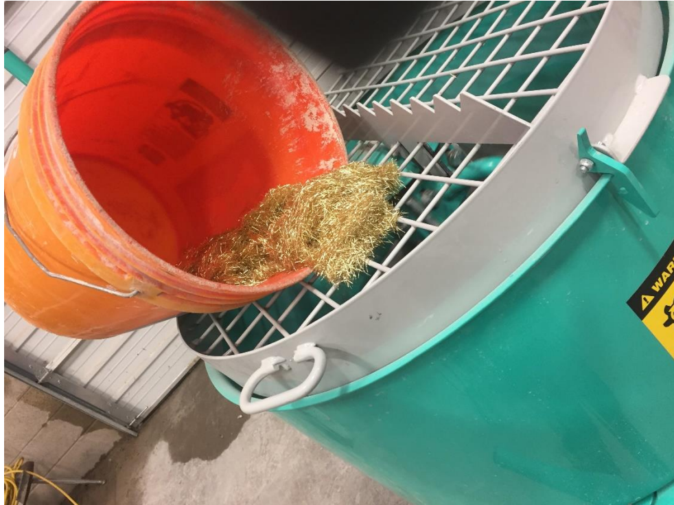
Figure 91. Steel fibers being added to UHPC mixture
