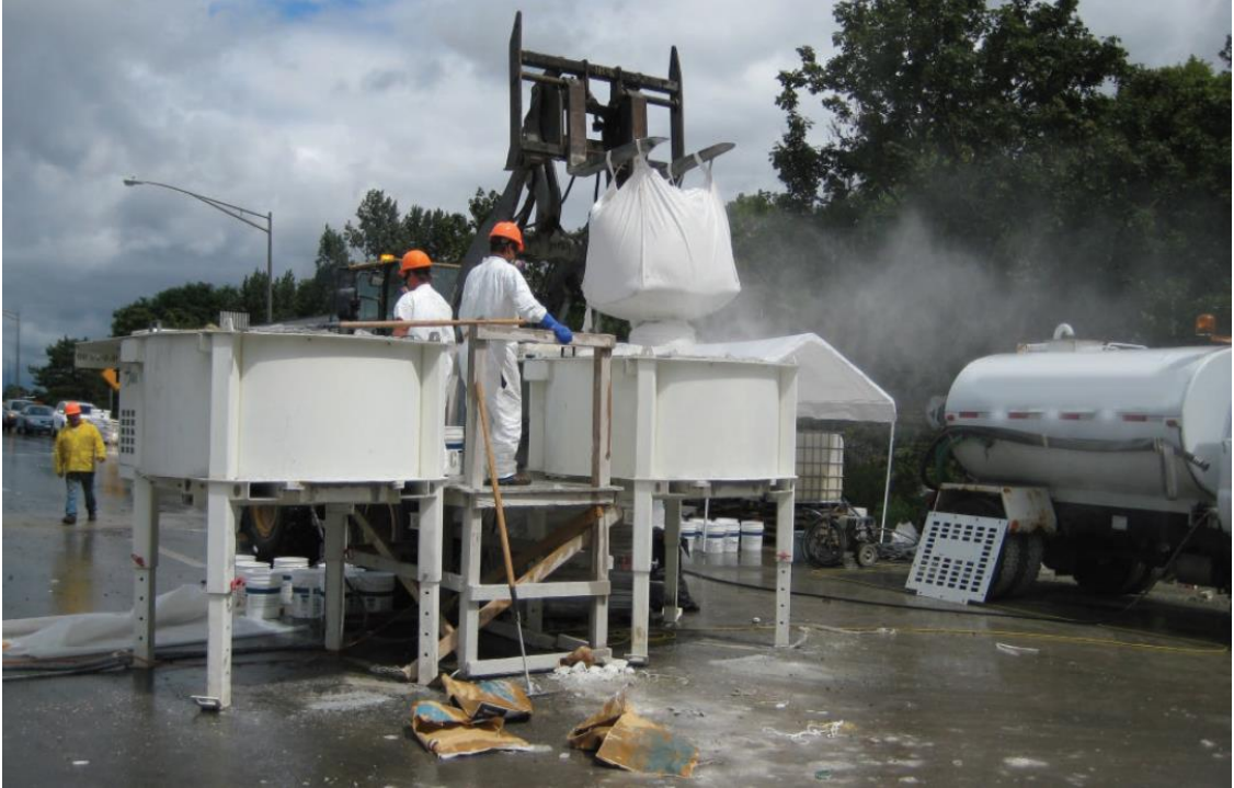
Figure 1. UHPC mixing operations (Graybeal 2014)
