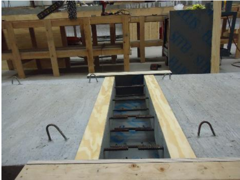
Figure 28. Rebar layout for UHPC joint
