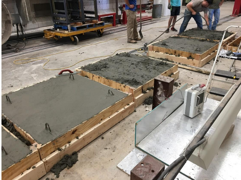
Figure 95. Slab panels during finishing process
