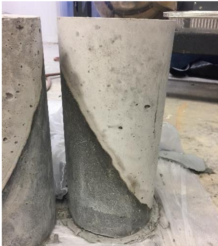
Figure 24. Composite slant shear specimen after curing
