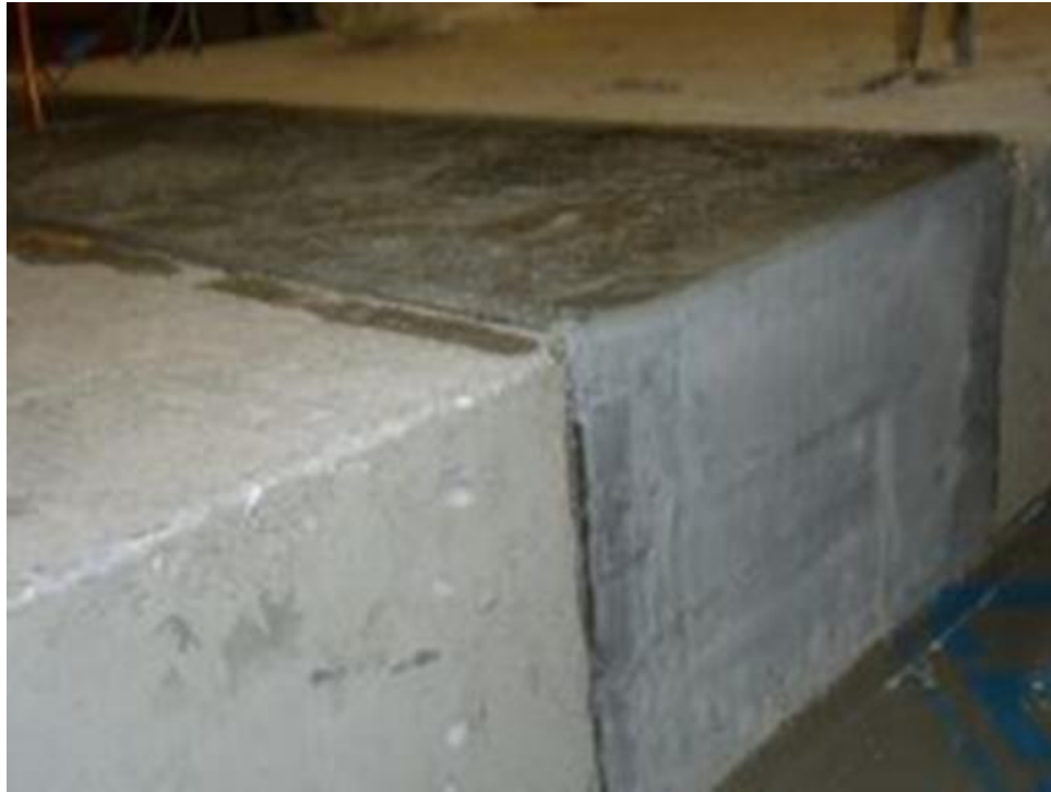
Figure 29. Completed UHPC joint after curing
