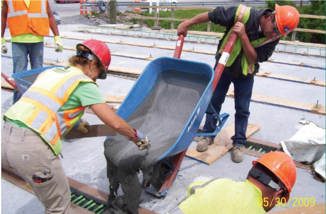
Figure 2. UHPC placement into longitudinal connection (Graybeal 2014)
