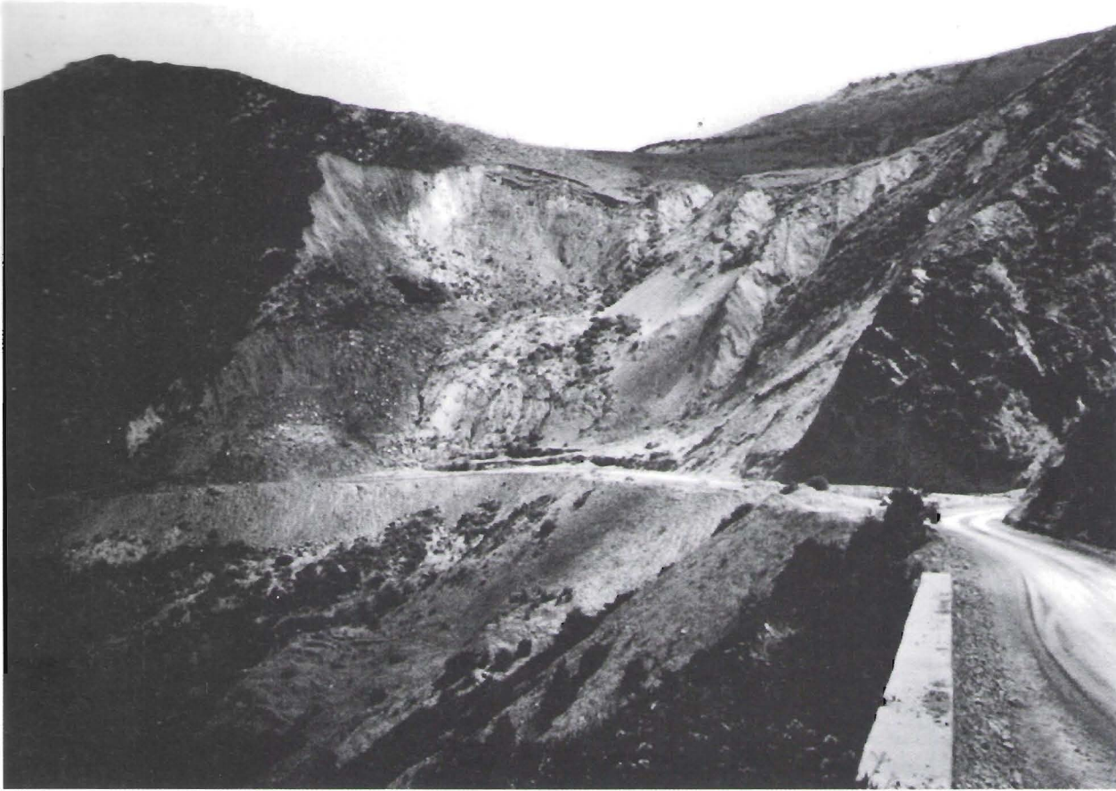
Figure 4. Slump blocks at the top of the active slump/earthflow that is crossed by the Chicoana-Cachi highway.
