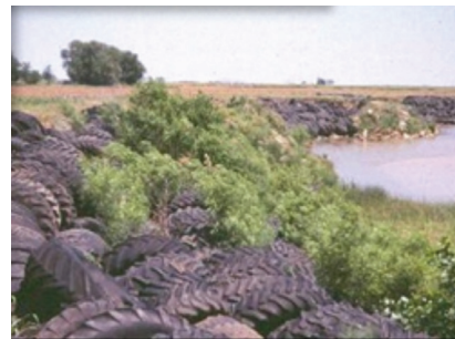
Figure 5. Concrete channel lined with riprap held in place with gabions in Stillwater, OK (A). Tire riprap along the Red River and concrete chunk riprap (B and C).
