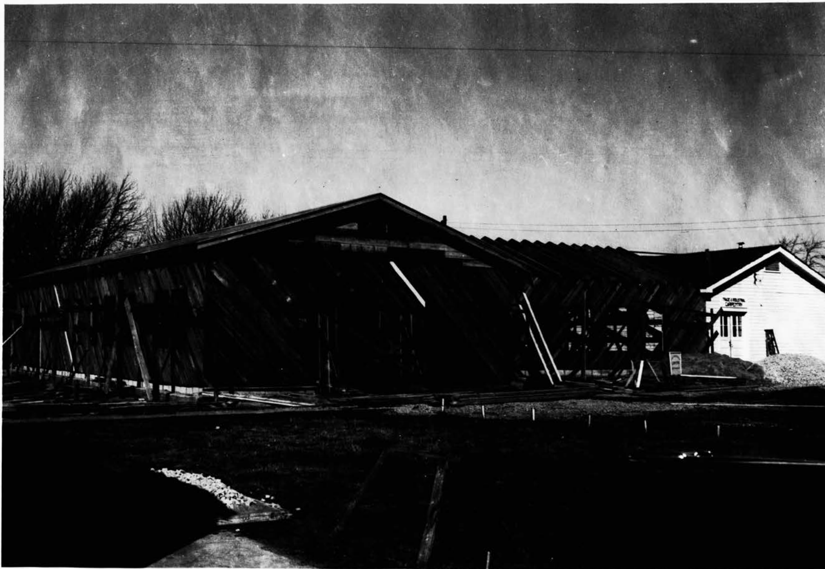
HOME ECONOMICS BUILDING Broken Arrow, Oklahoma
