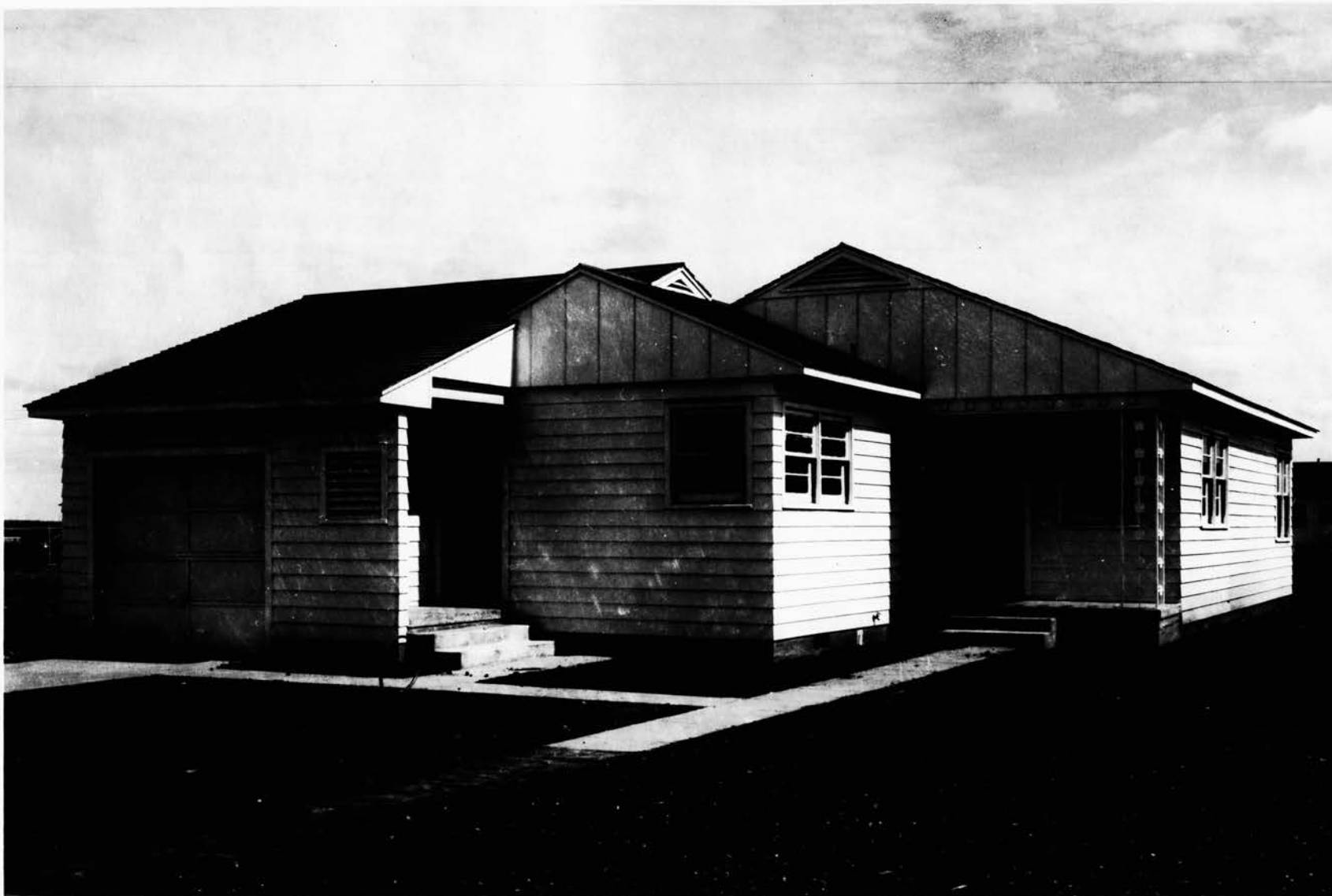
FIVE ROOM HOUSE Hobart, Oklahoma
