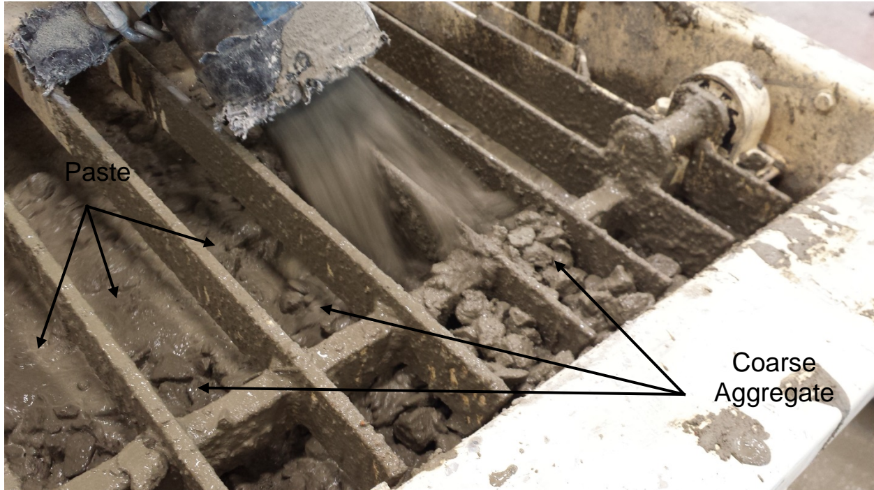
Figure 5-15 Coarse aggregate exiting the pipeline and showing segregation.
