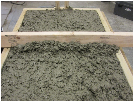
Figure 2-4: The concrete is leveled with a board
