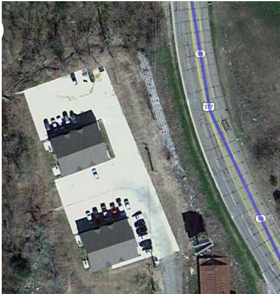
Figure_APX_B 3. Ariel shot of problematic Area after fix (note Gabion Walls on left side of road).
