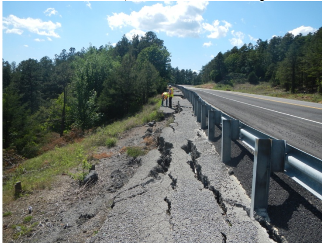
Figure_APX_B 21. Route 271, after Talimena state park Looking north. Project team is measuring water table depth in monitoring well.
