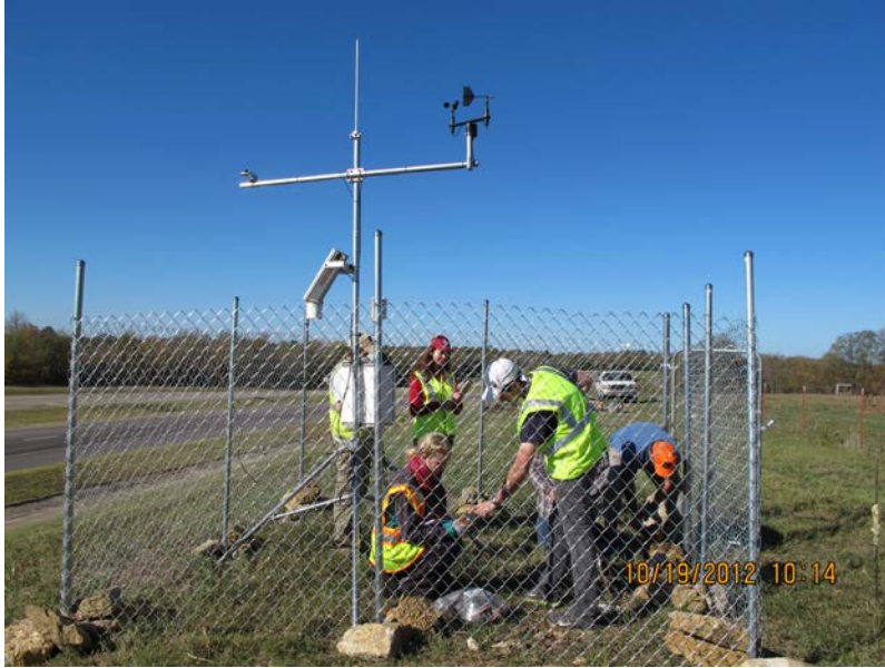
Figure 10. Weather Station Installation on the Slope.
