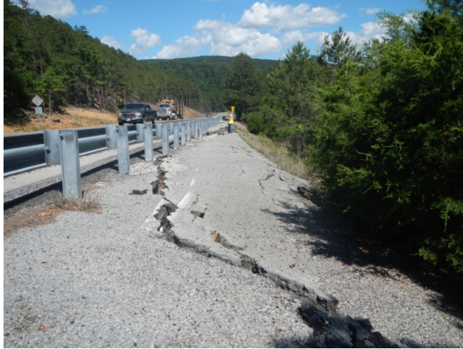
Figure_APX_B 20. Route 271, after Talimena state park Looking south.
