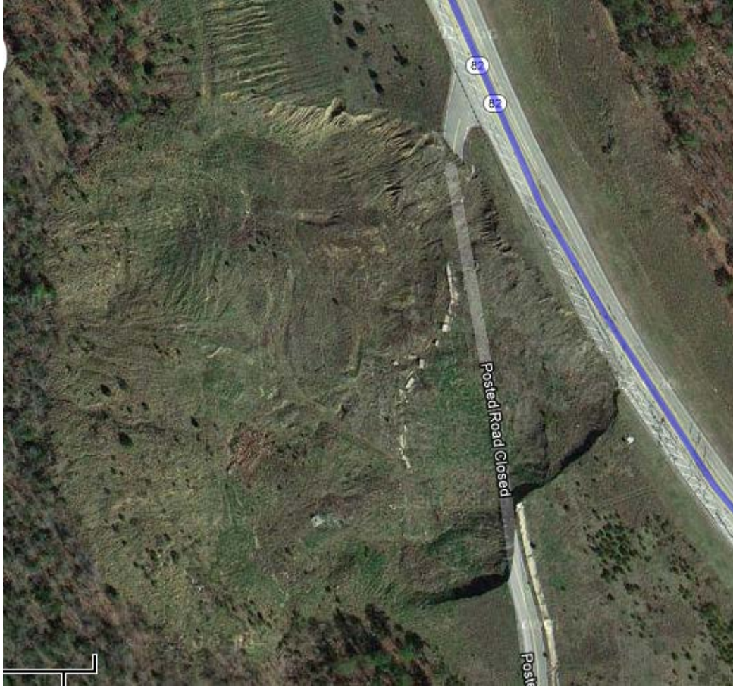
Figure_APX_B 26. Current satellite photo of the landslide mass.
