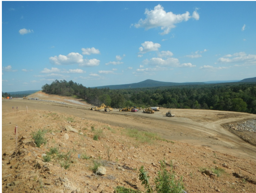
Figure_APX_B 24. Repairing the slide.
