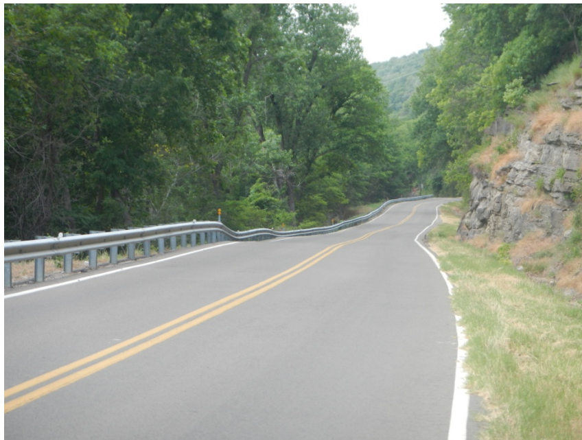
Figure APX_B 37. Looking toward Fort Gibson Dam, slide is on left (west).
