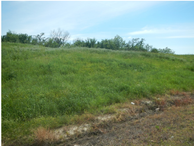
Figure_APX_B 15. Can see the headscarp here as a change in vegetation cover.
