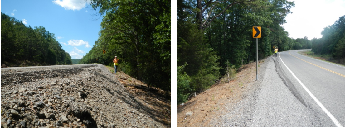
Figure APX_B 19. Shoulder pavement overlays.
